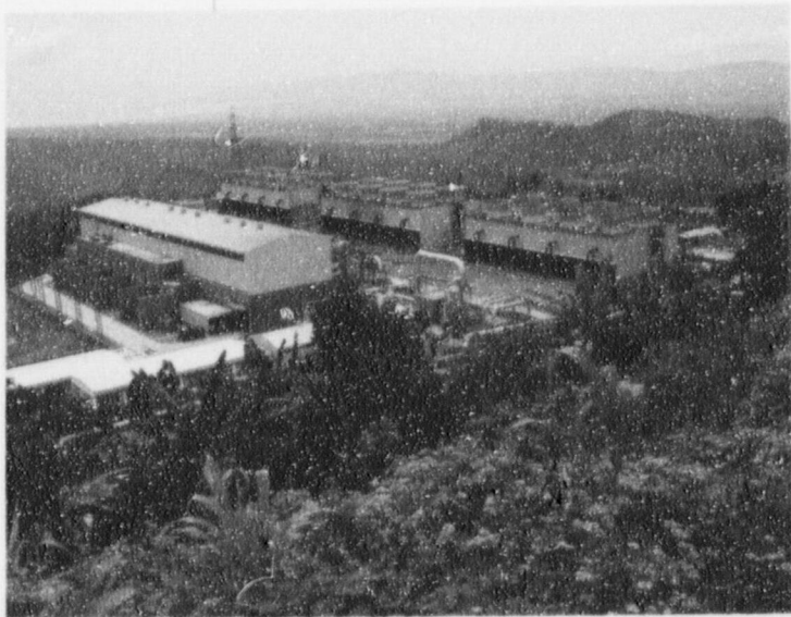
CalEnergy's Malitbog geothermal power project supplies much-needed electricity to the island of Leyte, Republic of the Philippines.
