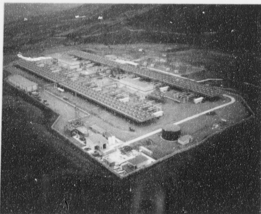
The first CalEnergy Philippine power project to receive revenue was the Upper Mahiao geothermal project located on the island of Leyte.
