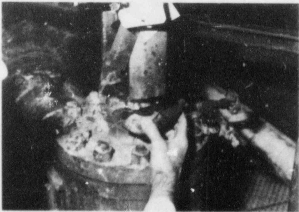
Figure 6.39 Closeup of FCV-457 Yoke Damage
