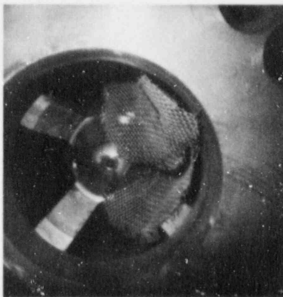
Figure 5.1-1 Damaged Full-Flow Filter Screen (View Looking Up Into Reactor Vessel)
