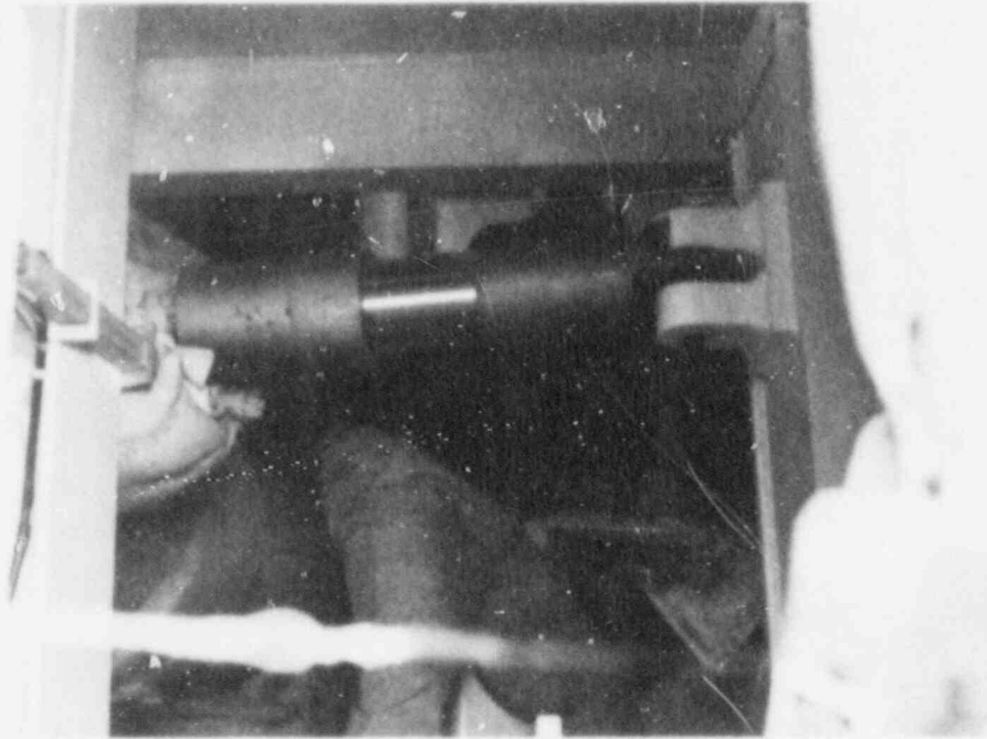
Figure 5.1-2 Feedwater Pipe Shock Suppressor (FW-9012-HL 5005) Attached to Reactor Coolant Pipe Rupture Restraint (RC1125R1)
