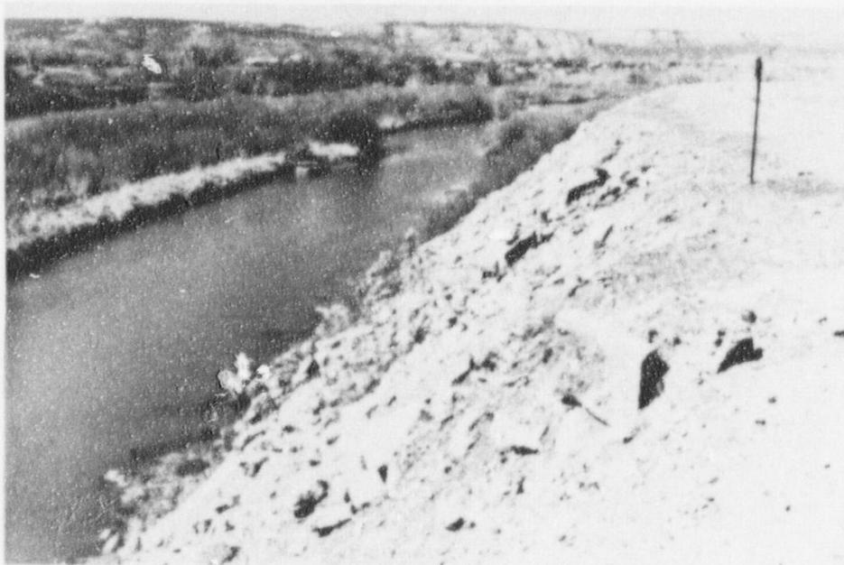
10. Concrete and building foundation riprap reinforcing south berm along Colorado River.
