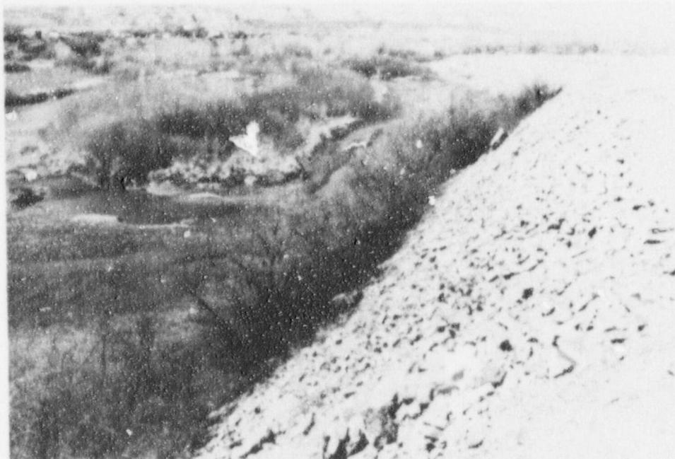
9. Brick riprap reinforcing south berm along Colorado River.
