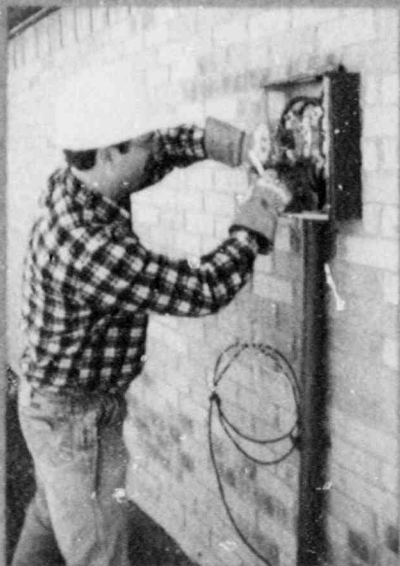
Distribution line work
