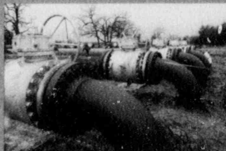
Gas pipeline addition
