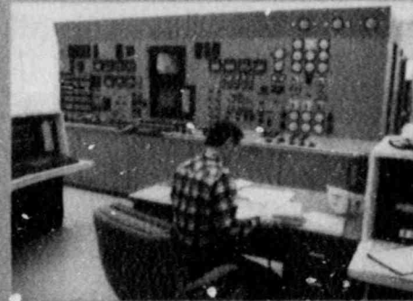
Control room at gas-fired plant
