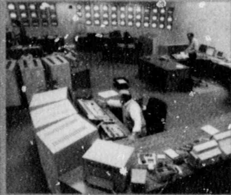
System operations center
