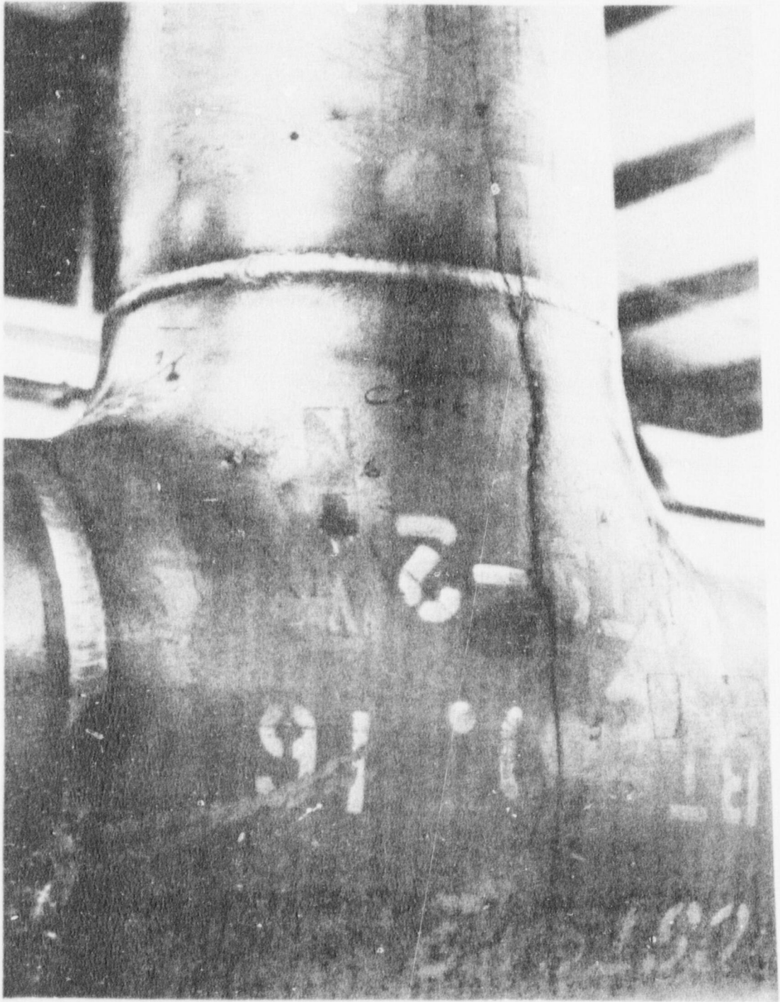
FIGURE 23. TEE, LOADED IN-PLANE (RUN), AT COMPLETION OF TEST (37)
