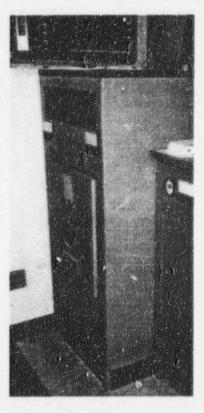
The battery chargers illustrated above are typical examples of rectifiers supplied by major U.S. manufacturers in the late 1960s and early 1970s. The same model La Marche charger is found at the Beaver Valley Unit 1 Nuclear Station (left), and at the Glendale Power Plant (right). The Glendale Plant withstood peak ground accelerations of about 0.30g in the San Fernando earthquake of 1971, and again in the Northridge earthquake of 1994.
