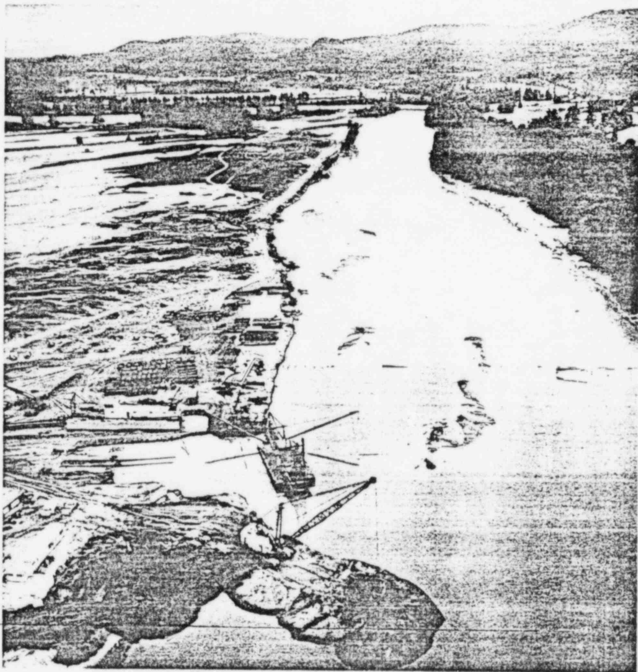
Pipeline dredges at launching site in the Cowlitz River. Islands in the shoaled riverbed and the mudfill outside the riverbank show impact of eruption mudflows.
