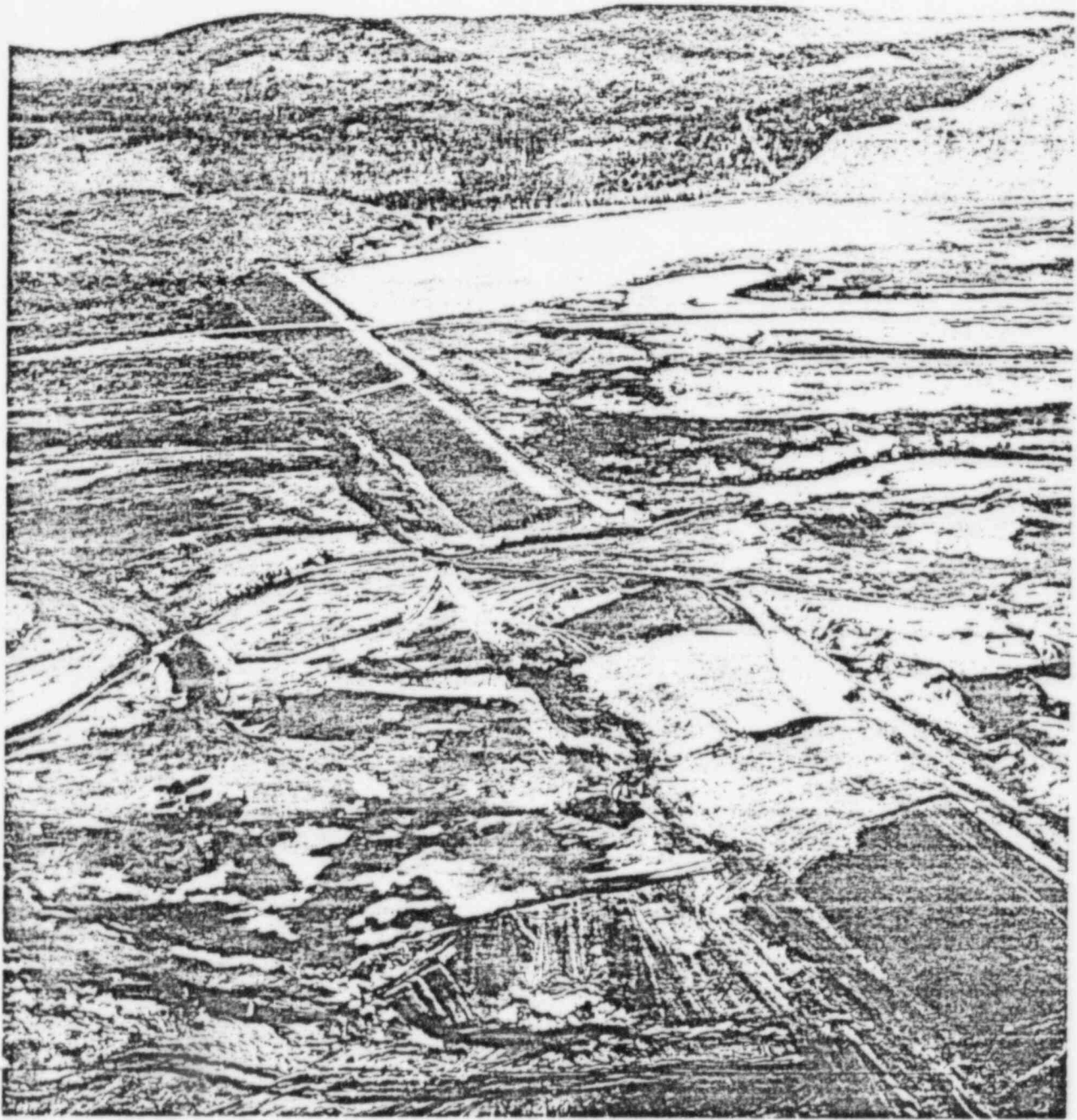
North Fork Toutle River debris retaining structure showing breached spillway caused by flood waters. New spillway under construction in foreground.
