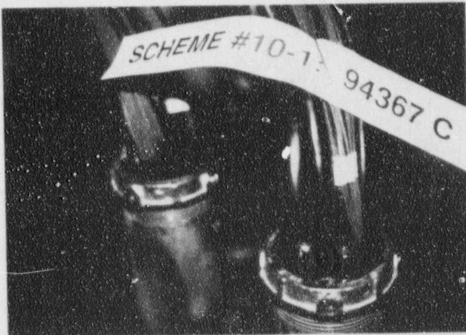
Foam/silicon seals installed at top of conduit runs.
