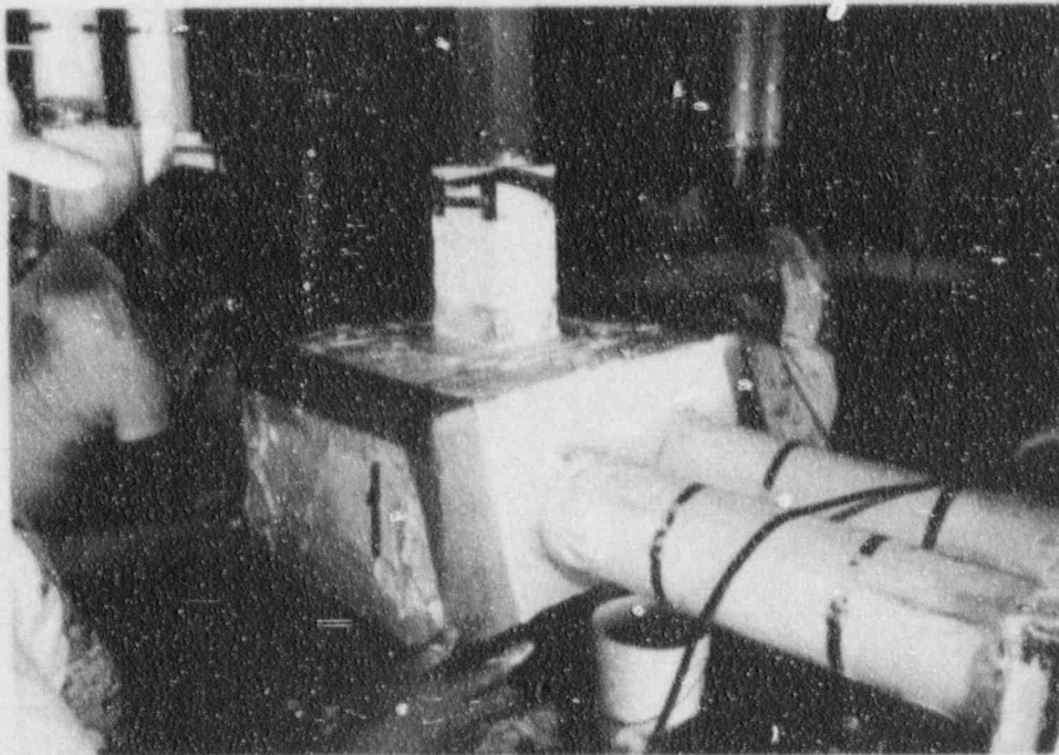
Stress skin edge treatment "upgrade" installed on junction boxes.
