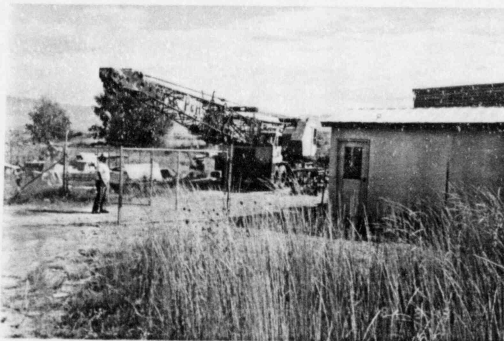
Front of Property Looking Northeast
