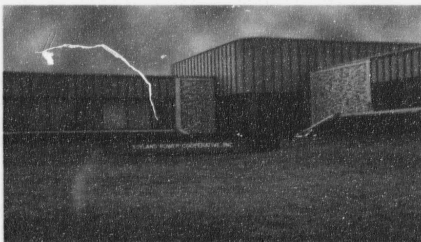
Soyland's main headquarters are located at 788 North Sunnyside Road in Decatur, Illinois.
