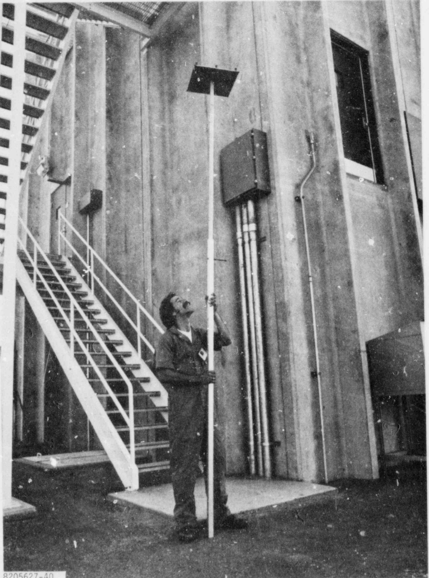
FIGURE 2-4. Special Fixturing Developed to Remotely Install the Protective Plate
