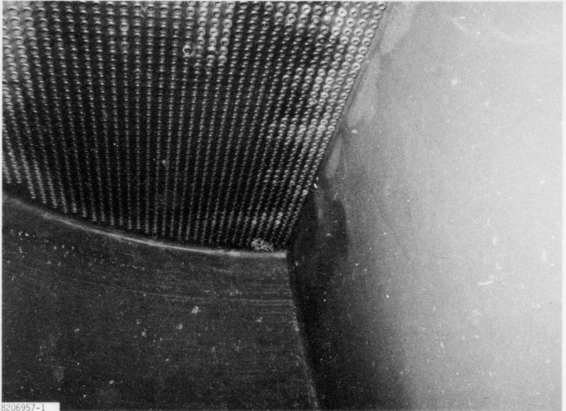
FIGURE 4-10. Hot Leg Surfaces Before Decontamination
