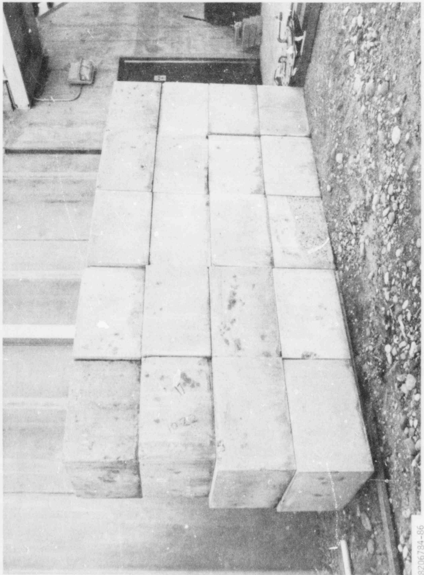
FIGURE 2-8. Concrete Block Shielding Wall Outside the Steam Generator Examination Facility
