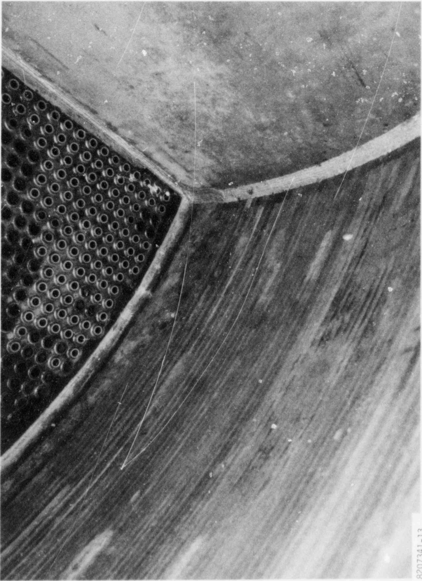
FIGURE 3-17. Cold Leg Surfaces After High-Pressure Water Rinse
