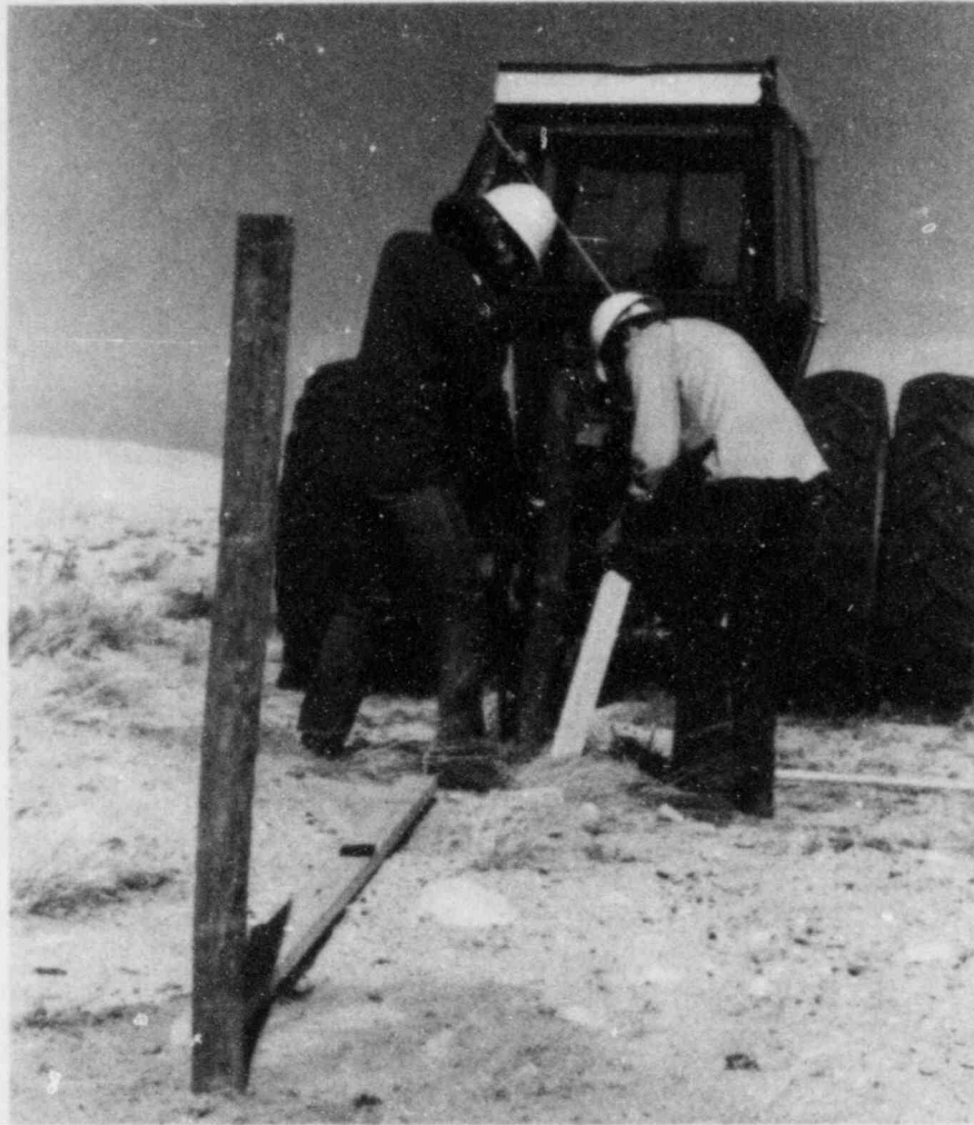
FIGURE 8. Wood Posts Tested as Supports for Selected Windscreen Test Panels
