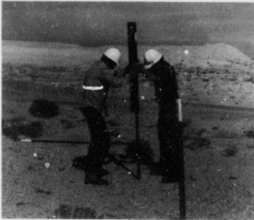
FIGURE 9. Steel Fence Posts Tested as Supports for Selected Windscreen Test Panels
