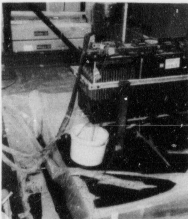
FIGURE 8 Simulated Electrolyte Leaking from a Cracked Battery Cell Case
