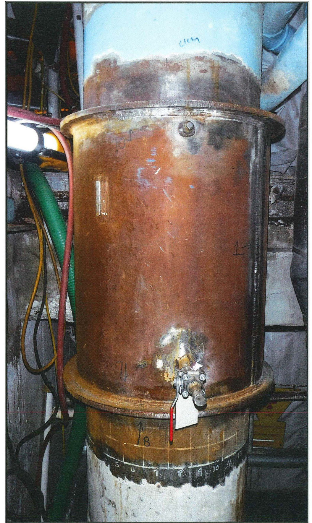
PM Cap Installed (Looking South)
