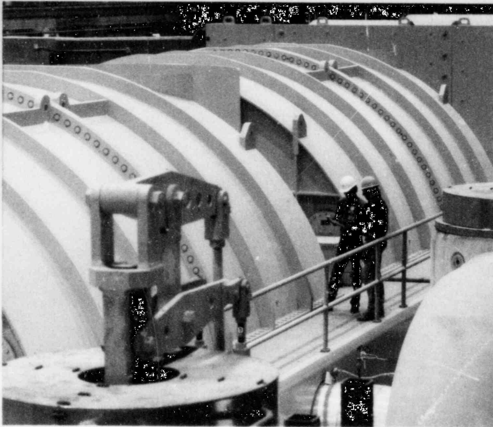
The Unit No. 1 turbine-generator will convert the steam produced by the reactor into electricity. The turbine-generator is 208 feet long and is designed to produce 1,100,000 kW of electricity.
