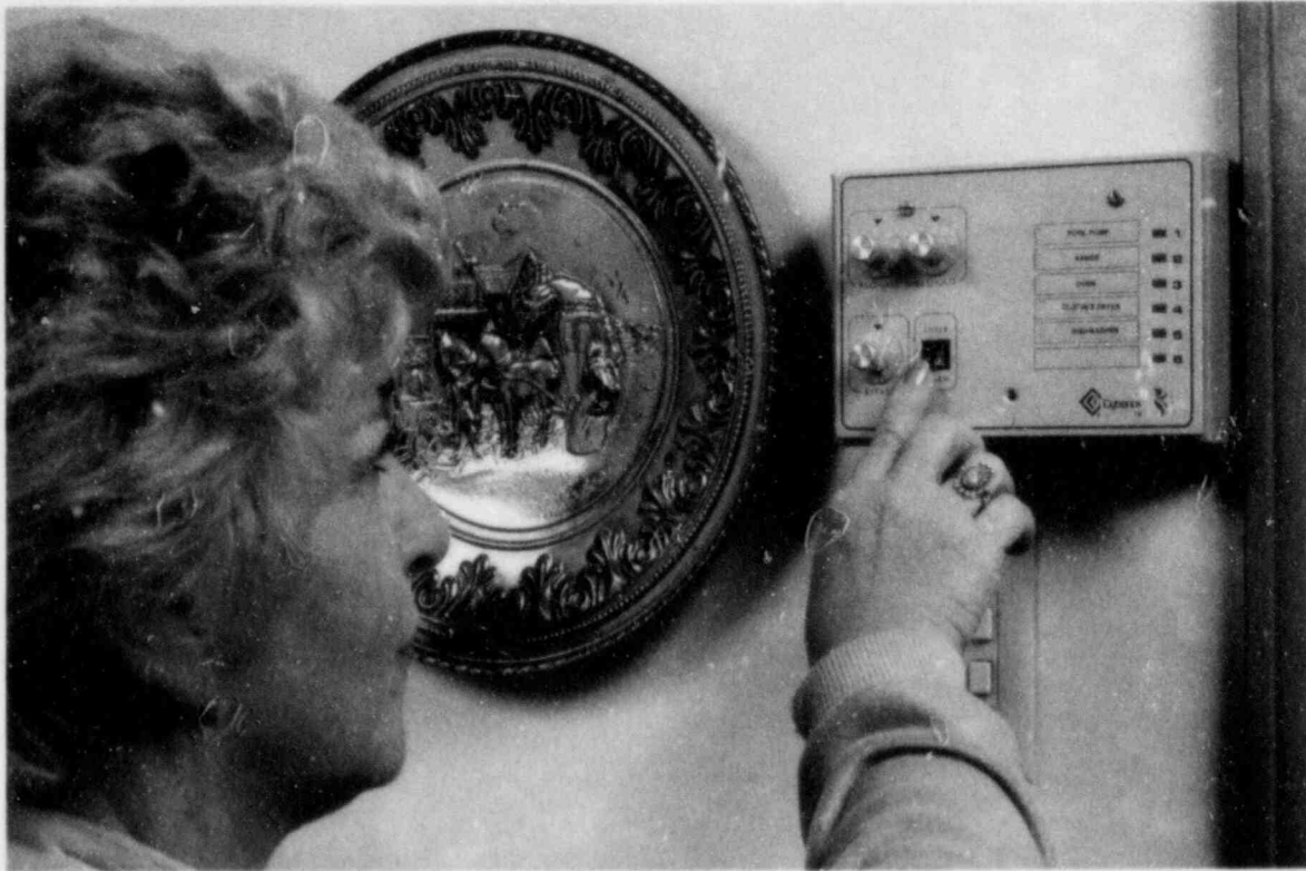
This load management panel controls major appliances in a customer's home to avoid heavy usage during hours of peak demand on the PSE&G system.
