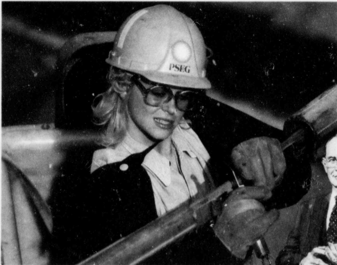
Wendy Schneck, Line-woman — Grade 2, rebuilds a pole top to prepare for conversion from 4KV to 13KV. Higher voltage will provide greater load capacity in the area and increase system efficiency.
