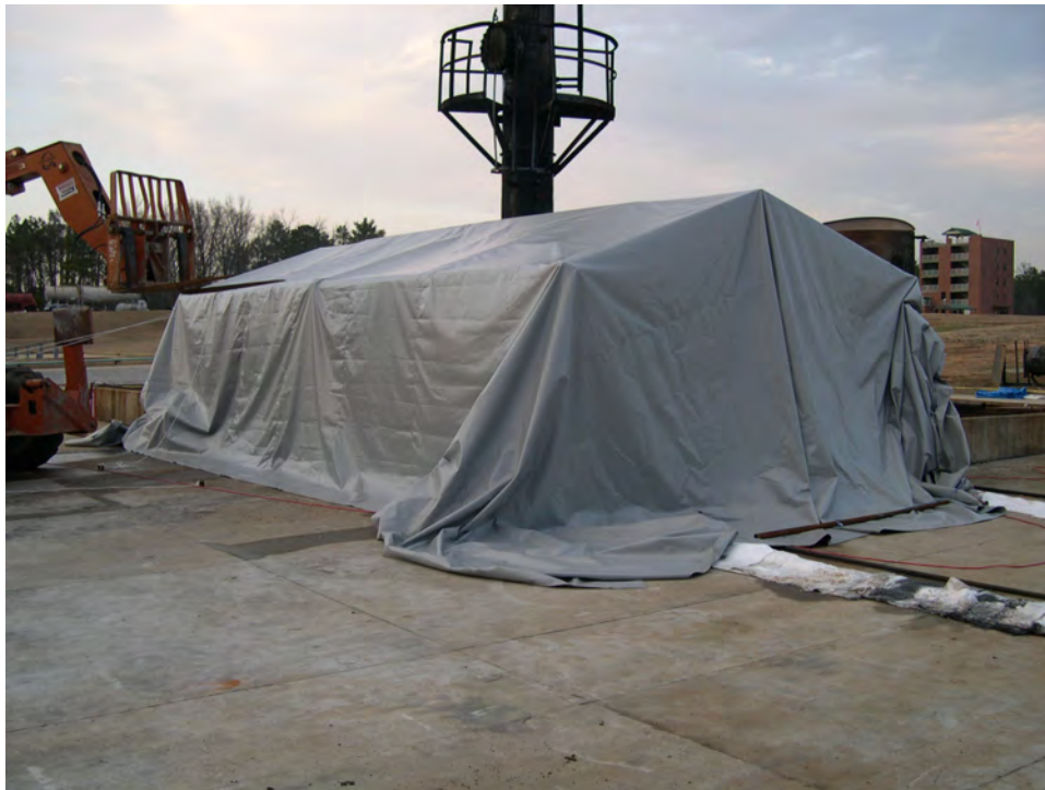
Figure 3-34 Test Article Under Tent to Maintain Temperature Overnight
