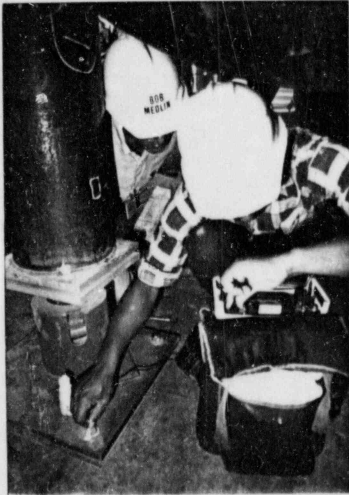
Photograph 3.1.5 Observation of UT measurements used to determine expansion anchor length.
