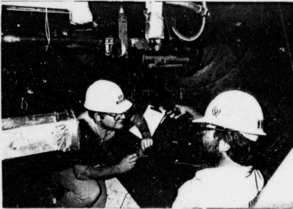
Photograph 3.4.1 Typical dry film thickness check on the containment plate.
