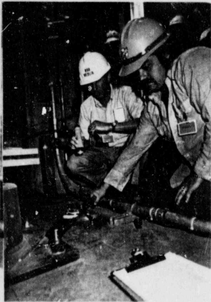
Photograph 3.1.3 Observation of torque applied to expansion anchor.
