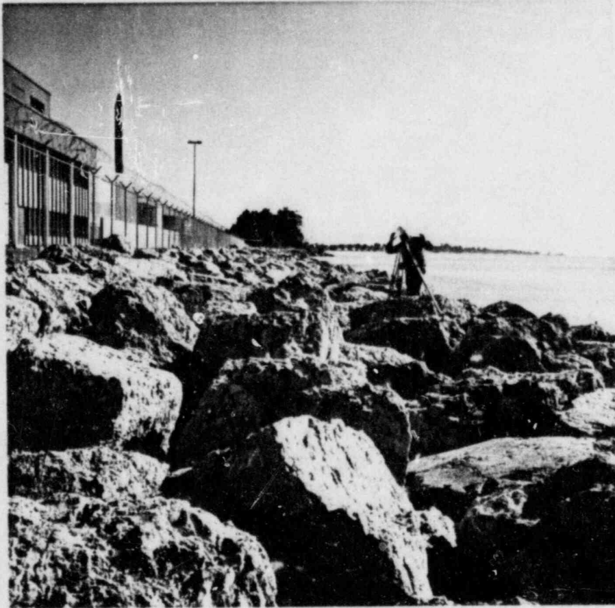
Photograph 3.2.5 Physical survey of shore barrier.
