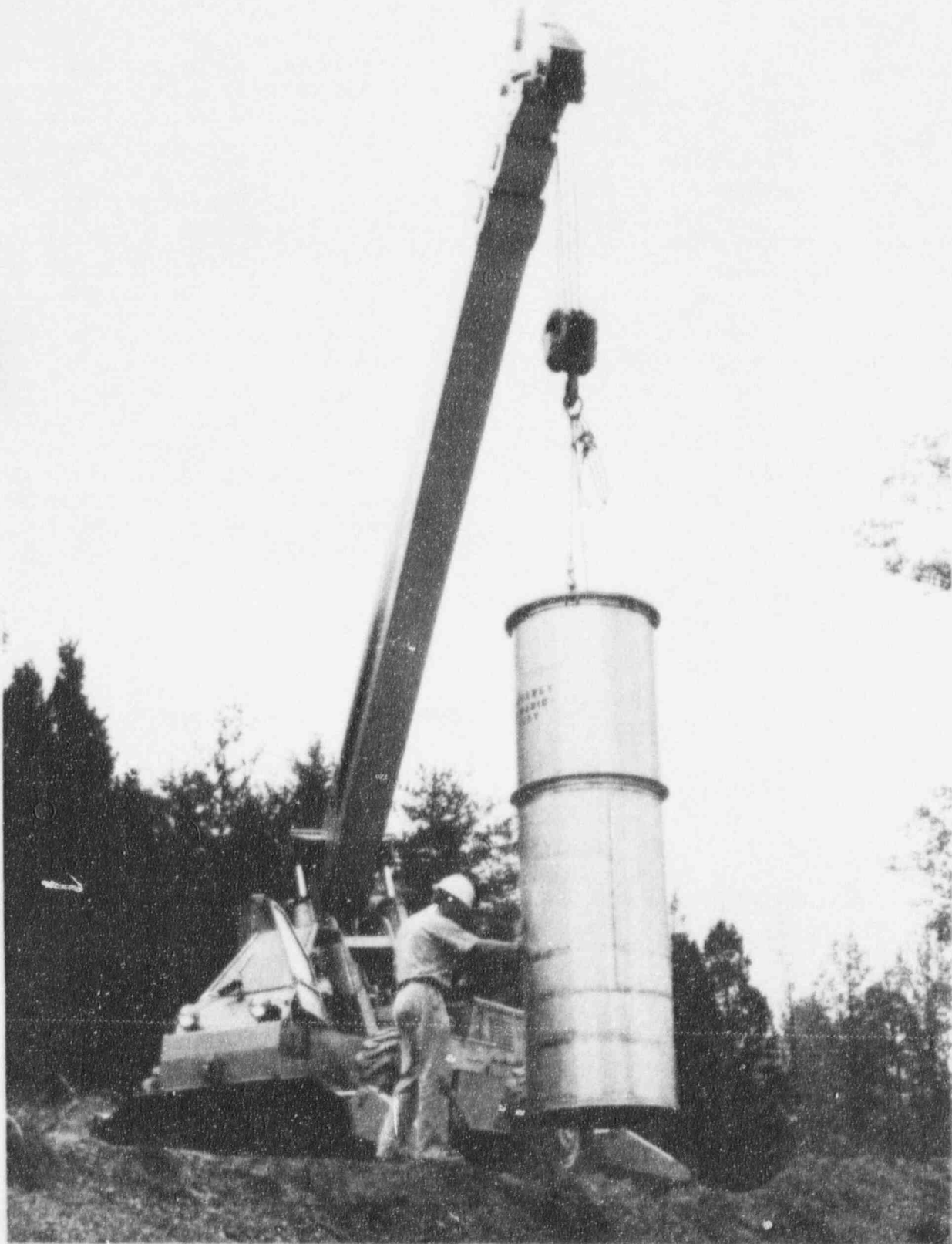
Figure 6. Unfilled lysimeter vessel being lowered into position at ORNL.
