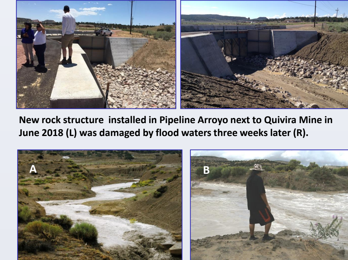
New rock structure installed in Pipeline Arroyo next to Quivira Mine in June 2018 (L) was damaged by flood waters three weeks later (R). Flood waters in Pipeline Arroyo next to the Quivira Mine (A) inundated a crossing on Pipeline Road one-half mile north of the UNC tailings dam in 2012 (B). These points are shown on the 2011 photo montage to the left. (Photo credits top: Paul Robinson, Edith Hood; bottom: Terry Keyanna.)
