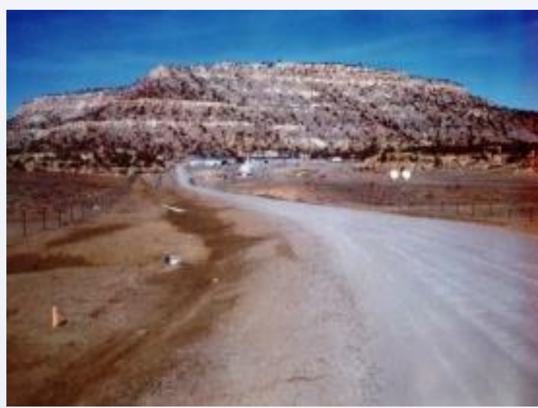
Red Water Pond Road leading to the Kerr-McGee Church Rock I Mine, 1972. Mine headframe seen in rare. The road bed was made with mine waste, which was excavated and removed 40 years later in 2012. (Photo credit: Tony Hood)
