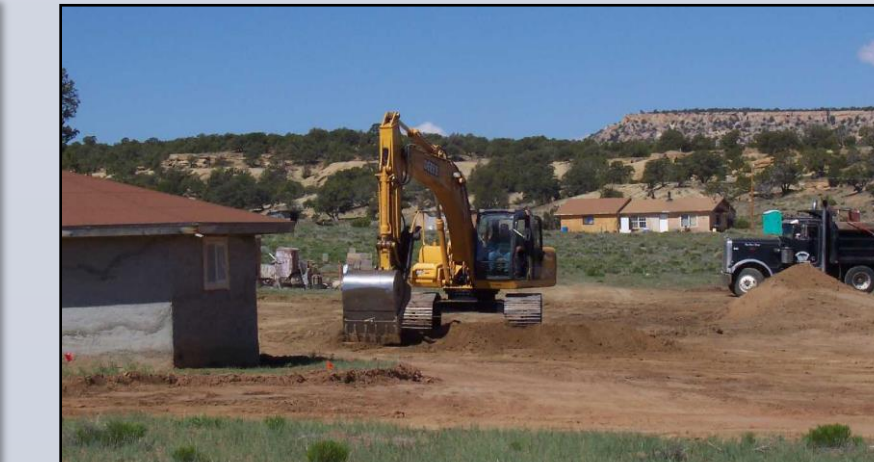
Backhoe removes soil around hogan, May 2007
