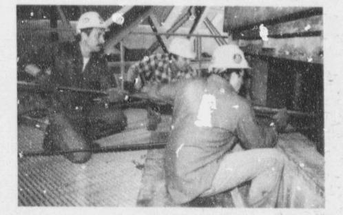
Plant Merrow Mechanics (from left) Tommy Mills, James Woods, and Don Harvey change out air preheater baskets located in the combustion air "ath. Weighing up to 300 pounds apiece, the baskets act as heat exchangers to help improve combustion efficiency in the boilers. and install replacement tube sections. To reduce the potential for overheating and water circulation problems, rifled tubes were specified instead of the smooth bore of the original tubes.
