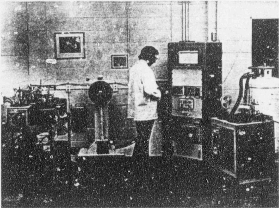
Figure: C-1. Charpy Impact Test System, Associated Constant Temperature Baths and Instrumented Charpy Impact Data Processing Equipment.
