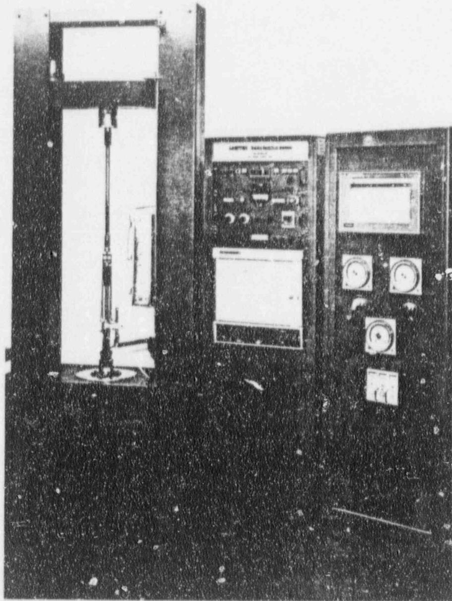
Figure: B-1. Tensile Test System with Control Console and Elevated Temperature Testing Equipment
