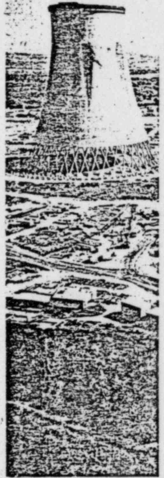
LIMERICK I is almost 80 percent complete and scheduled to begin producing power in April, 1985, provided the Nuclear Regulatory Commission approves its license.
