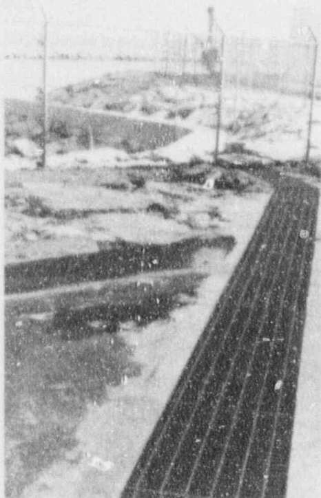
Plate 1. The 300 foot long Pilgrim Station, concrete screenwash sluiceway is molded from 18" corrugated metal pipe, and meanders over breakwater rip rap.
