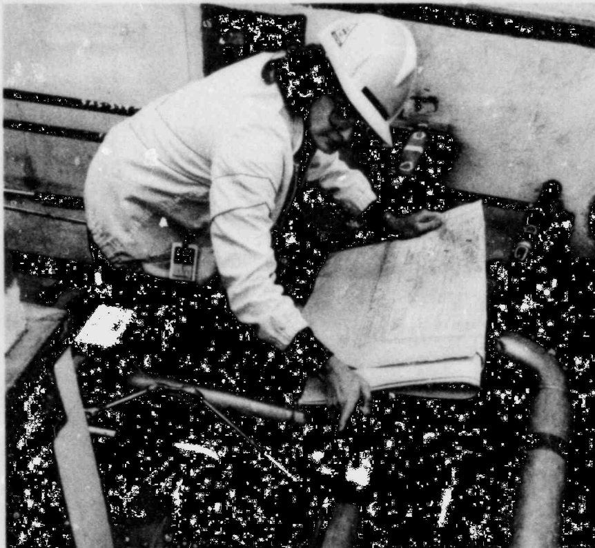
Ohio Edison employees are directly involved in construction progress at the Beaver Valley Power Station unit 2.
