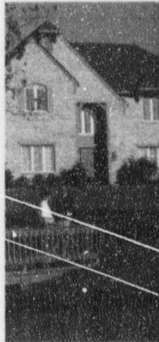
Many builders are installing high-efficiency, geothermal heating and cooling systems, called System:GT ® in new homes such as this one near Medina, Ohio.
