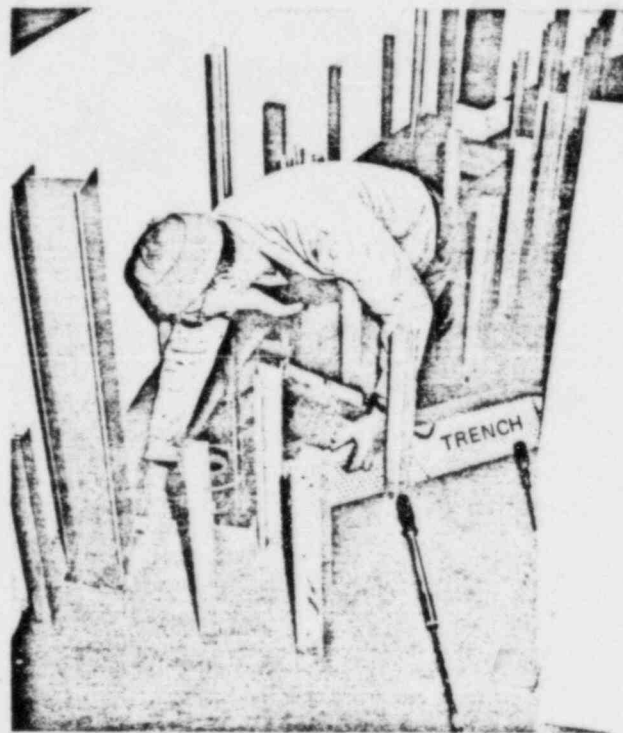
FIGURE 6 SUMP DURING CONSTRUCTION
