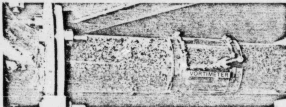
FIGURE 8 VORTIMETER ACCESS PORT
