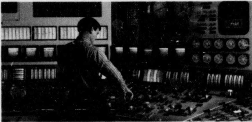
Duke's Marshall Steam Station was the most efficient coal-fired plant in the country in 1982. A Duke plant has led the nation in fuel efficiency 15 of the past 17 years.
