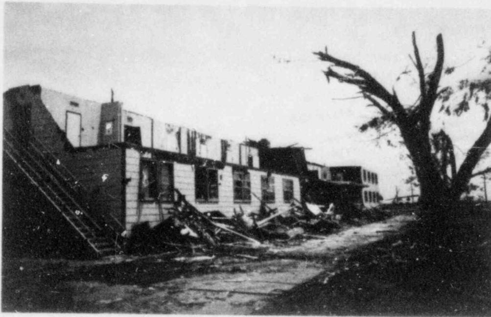
FIGURE 18. SEVERE-LOOKING DAMAGE TO WOODEN BARRACKS (most barracks lost their roofs and parts of second-story walls).
