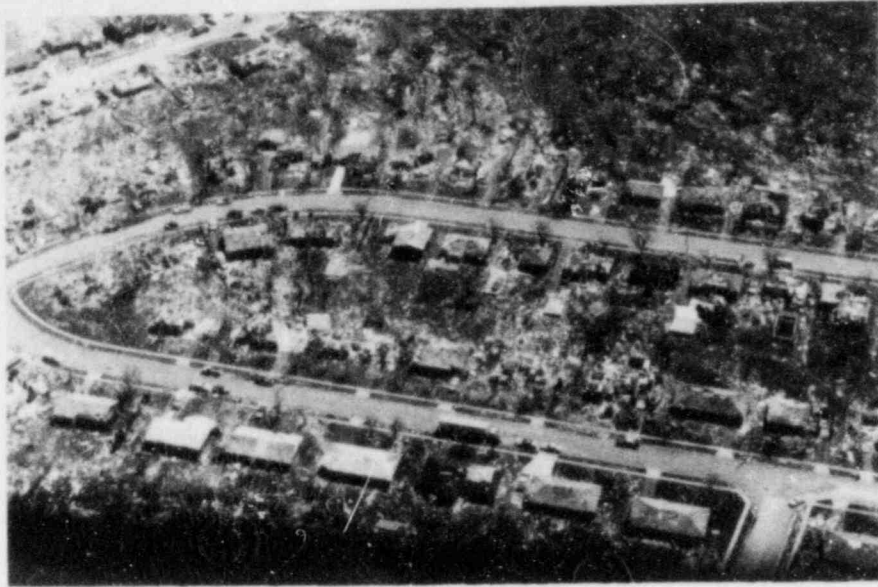
FIGURE 4. DAMAGE TO RESIDENCES IN XENIA, OHIO
