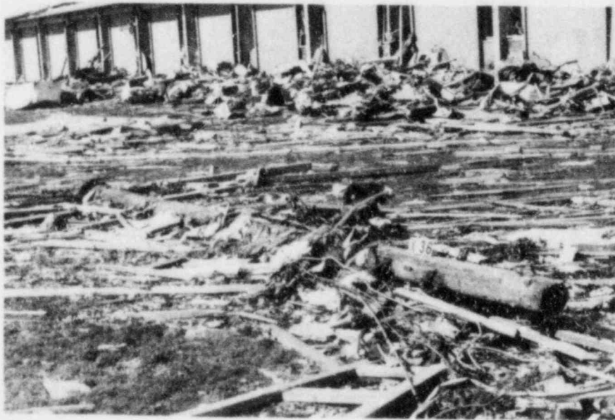
FIGURE 5. DEBRIS HAS COLLECTED AGAINST ARROW WOOD SCHOOL (when a structure interferes with flow of debris, it gives appearance of a swath)
