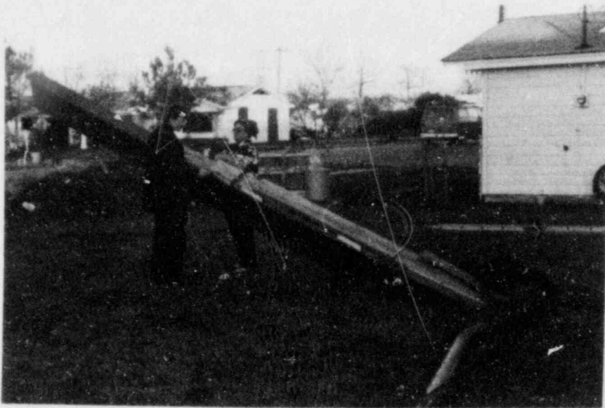
FIGURE 8. STEEL WIDE FLANGE BEAM TRANSPORTED BY BOSSIER CITY, LOUISIANA TORNADO
