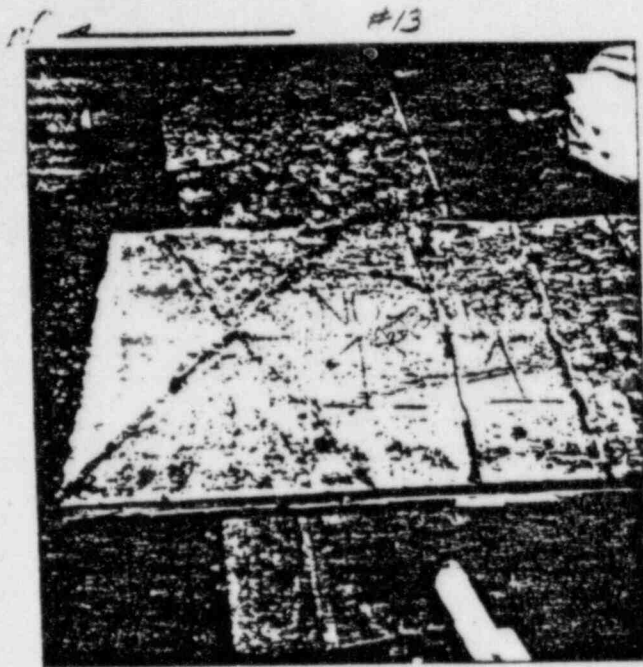
6/29/83 RATE No. 1 (NORTH END) CONCRETE CUT "X" PATTERN, 4 NIPPLES FINE RATE, WOOD BULKHEAD
