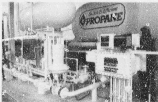
New truck docks were installed at the caverns in 1991. This enhancement doubled the loadout capacity to eight trucks per hour. The average load on each truck is 9,500 gallons.
