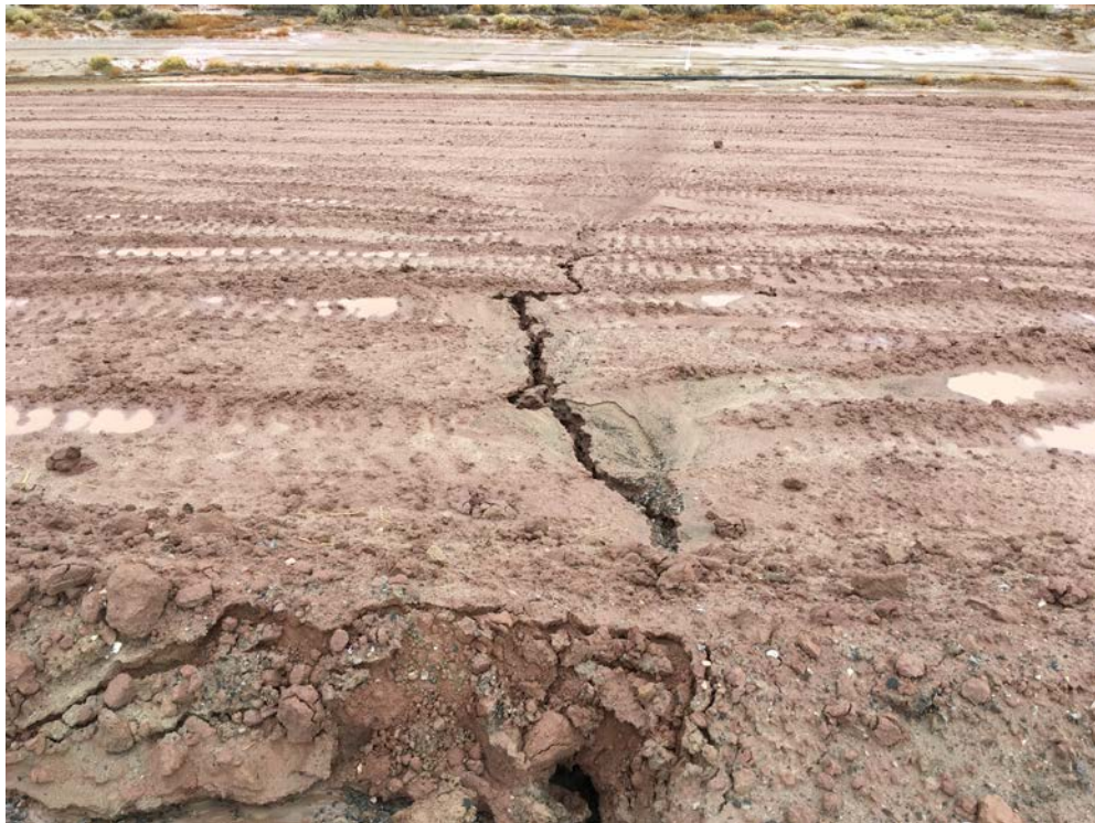
Photo 29: EP-1, rilling on the east embankment downslope
