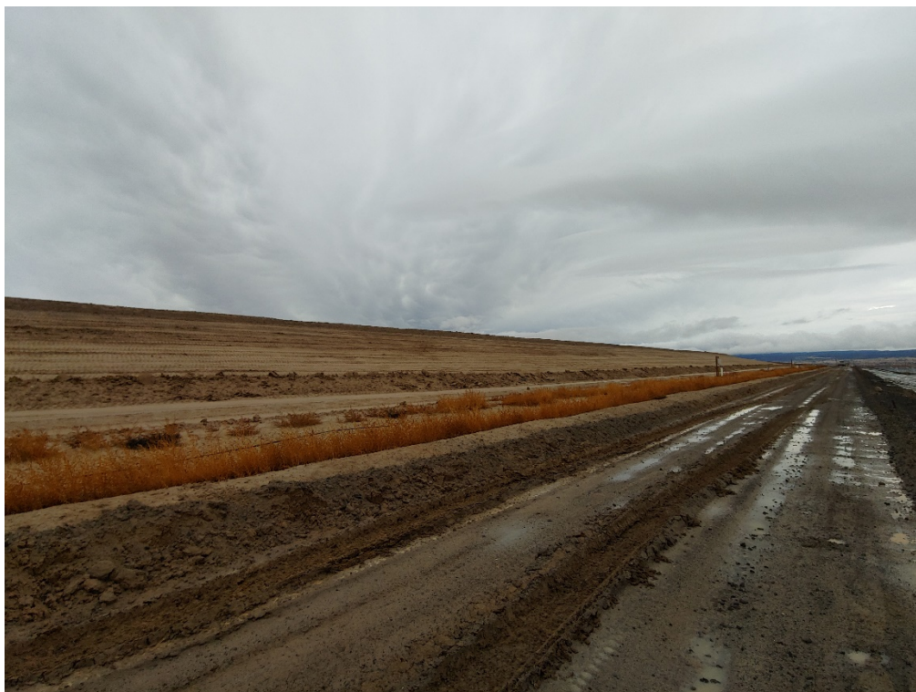
Photo 31: STP/EP-1, toe of slope along the south embankment
