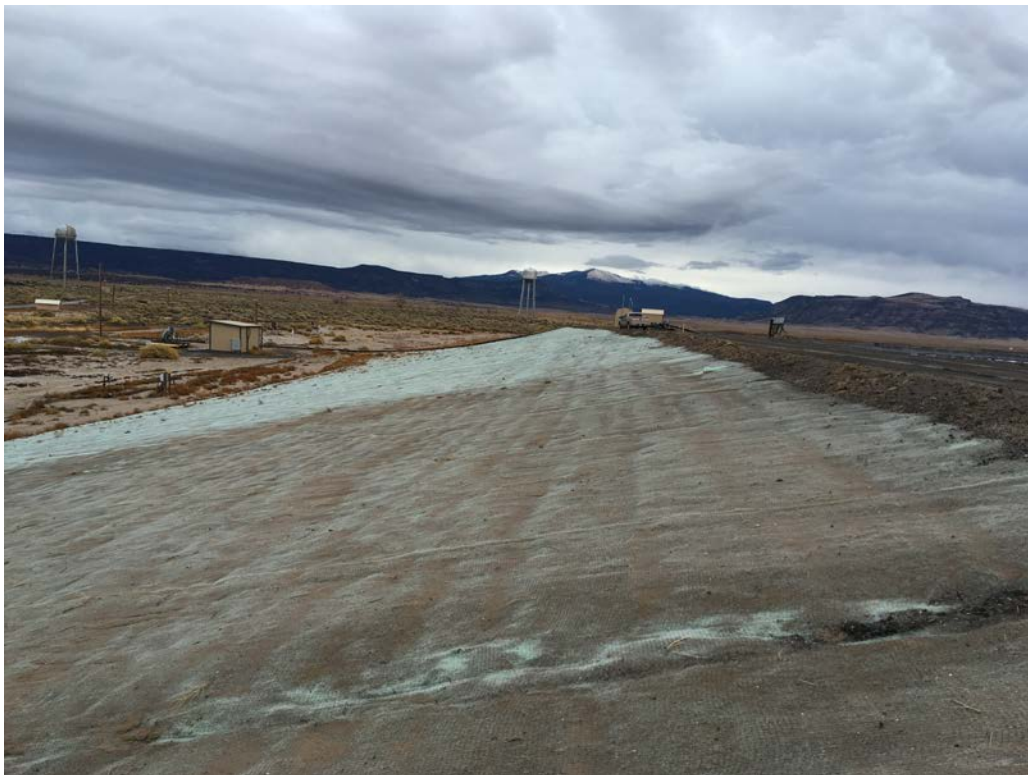
Photo 26: EP-1, erosion mat on the north embankment downslope
