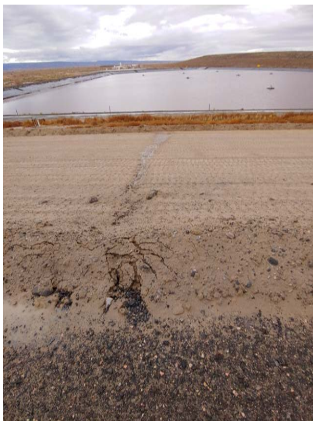
Photo 35: EP-1, rilling present on downslope of west embankment. Looking towards EP-2
