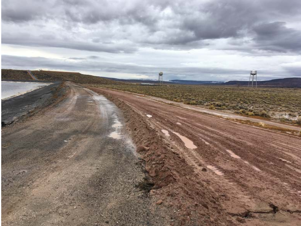
Photo 28: EP-1, erosion through crest safety berm and rilling on the east embankment downslope
