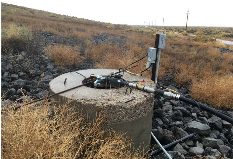
Photo 6: LTP, French drain/sump system at downstream toe of north side slope
