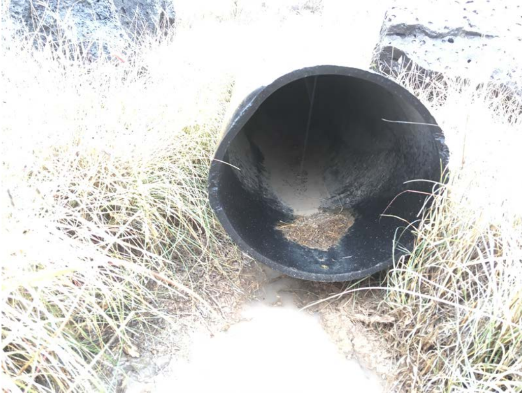
Photo 9: LTP, absence of water draining from downdrain on west slope
