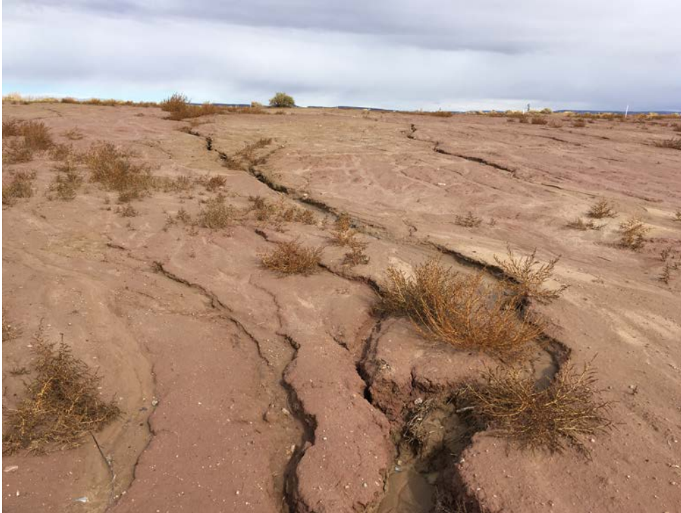
Photo 19: LTP, rilling on south side of top surface, adjacent to area regraded in 2019
