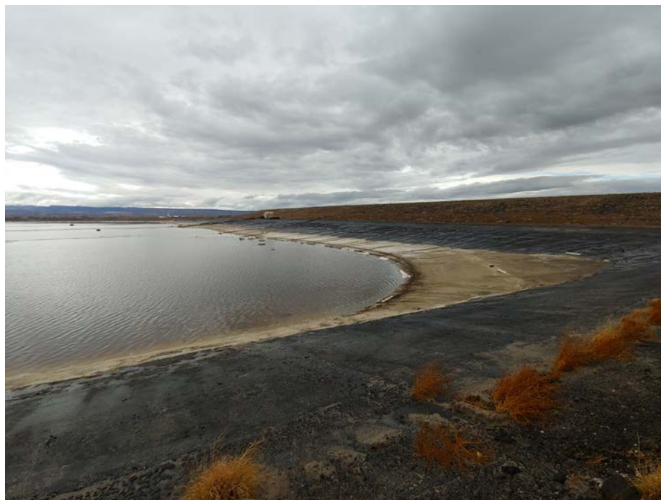
Photo 34: EP-1, general conditions of northeast corner, looking west
