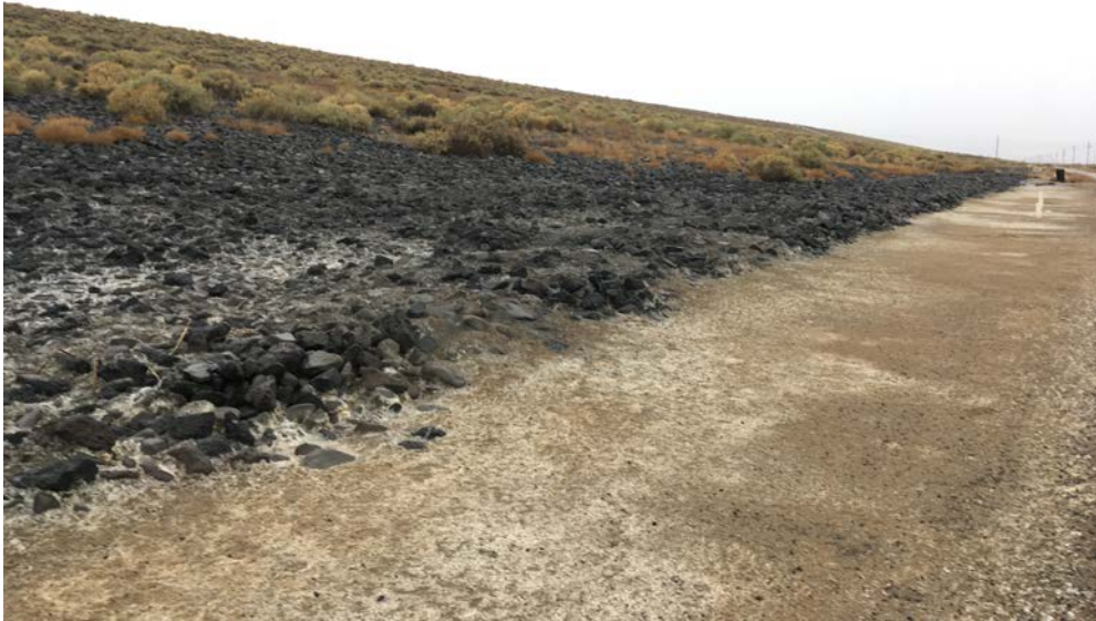
Photo 1: LTP, downstream toe along north side slope (looking west)
