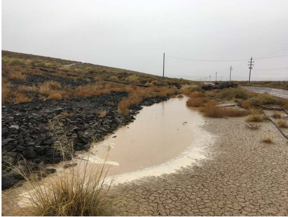
Photo 3: LTP, ponded water at downstream toe of north side slope
