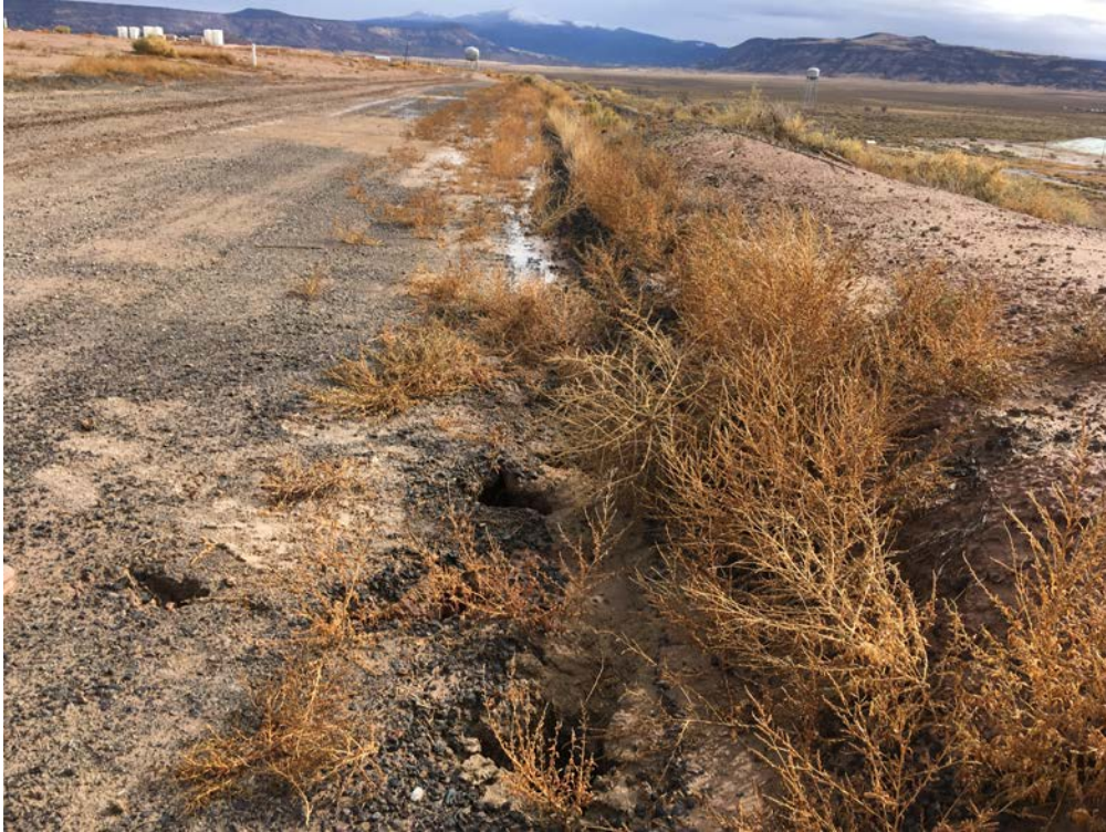
Photo 17: LTP, sinkhole extending to the east of downdrain #11
