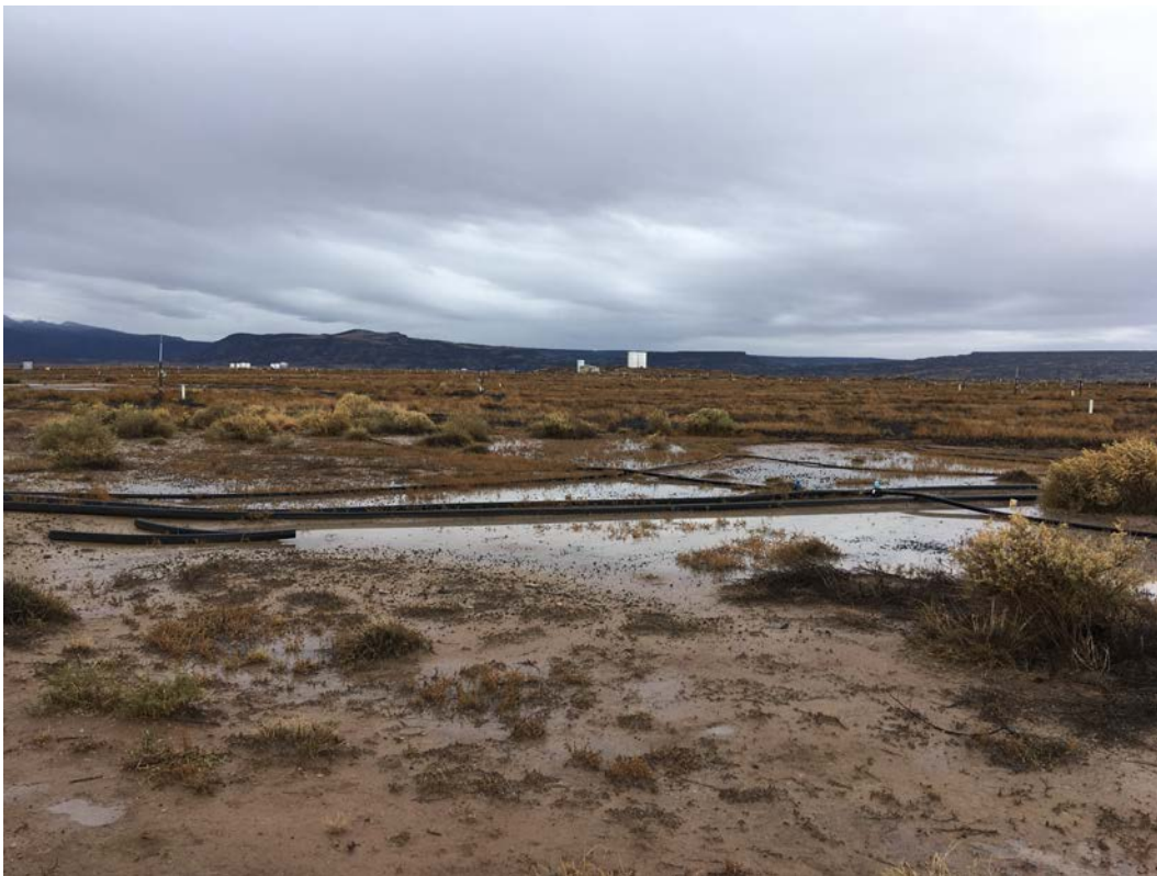
Photo 10: LTP, ponded water on top surface near the western edge
