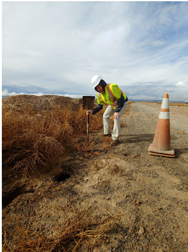
Photo 16: LTP, sinkhole near downdrain #11, shovel used to show approximate depth of hole
