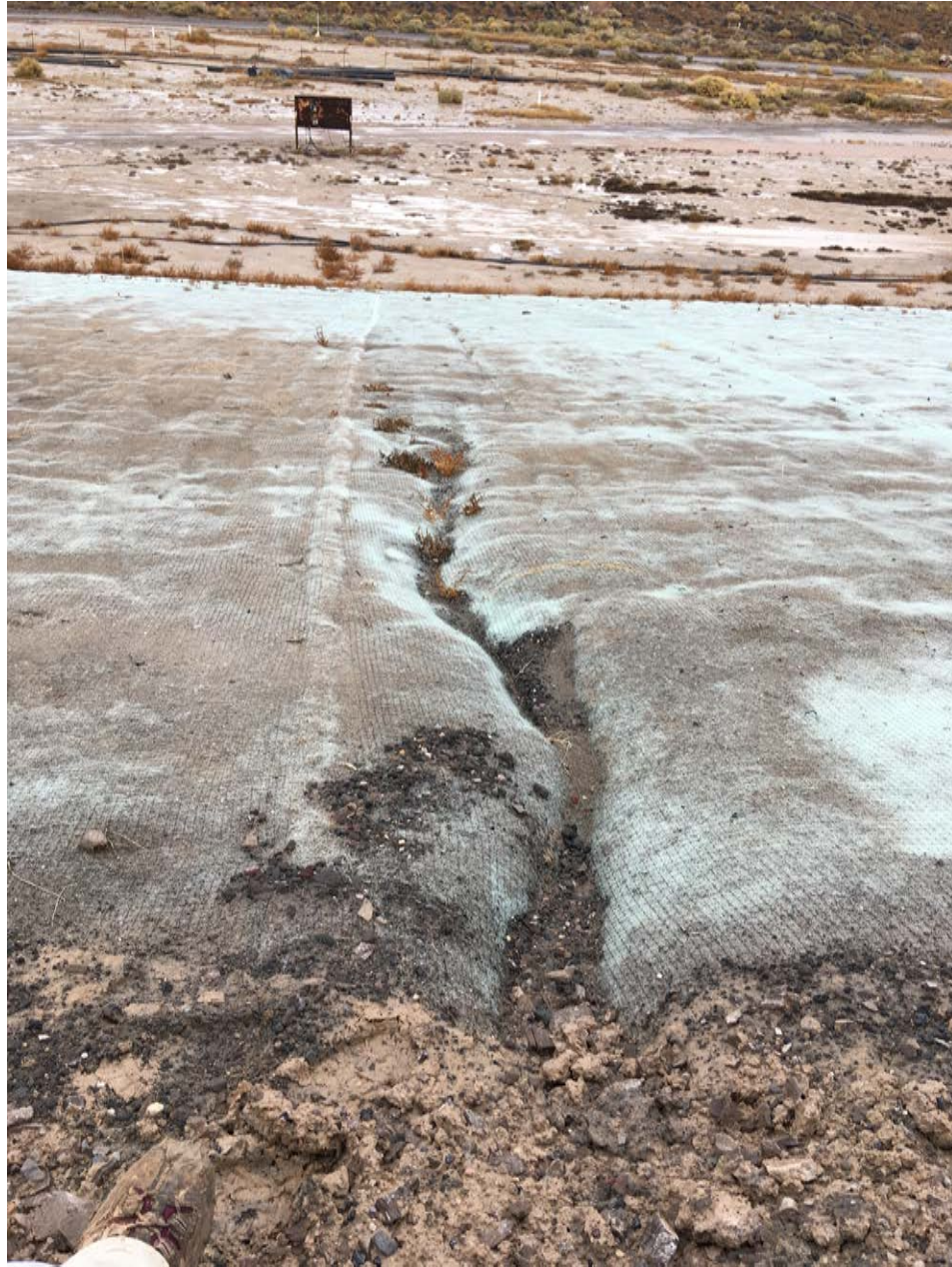
Photo 27: EP-1, rilling present underneath erosion mat on the north embankment downslope
