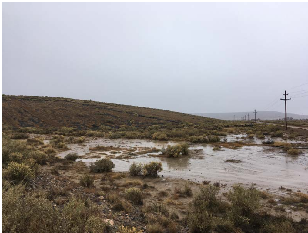
Photo 7: LTP, ponded water (from recent storm) at downstream toe of northwest corner of impoundment
