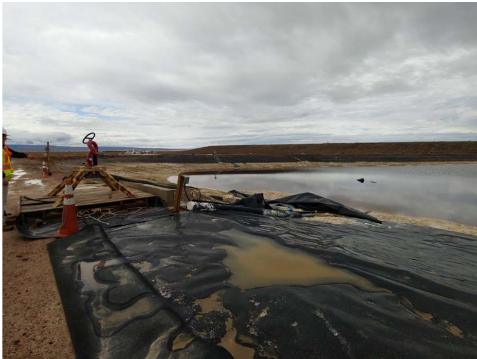
Photo 33: EP-1, location where WCP sediment being deposited to EP-1 along south embankment
