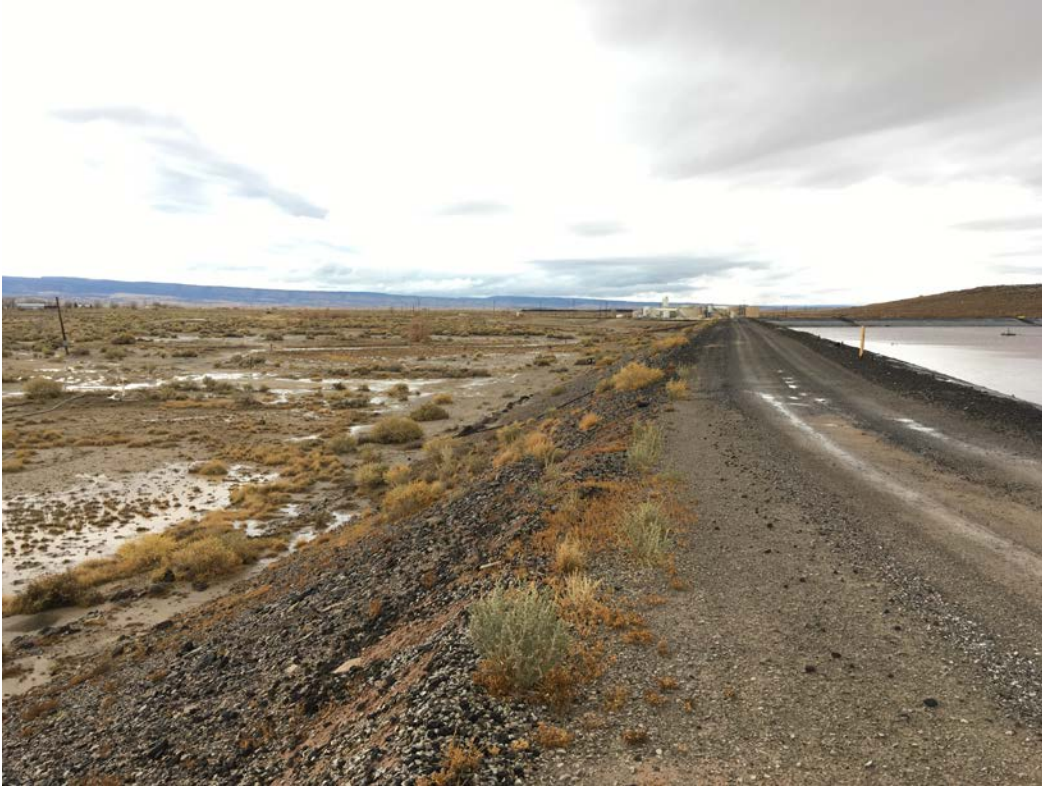
Photo 25: EP-2, downslope and crest road of the south embankment
