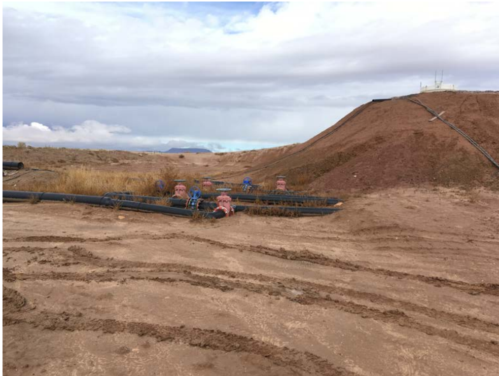
Photo 20: LTP, new pipes near zeolite system on east end. Partial repair of berm corner completed
