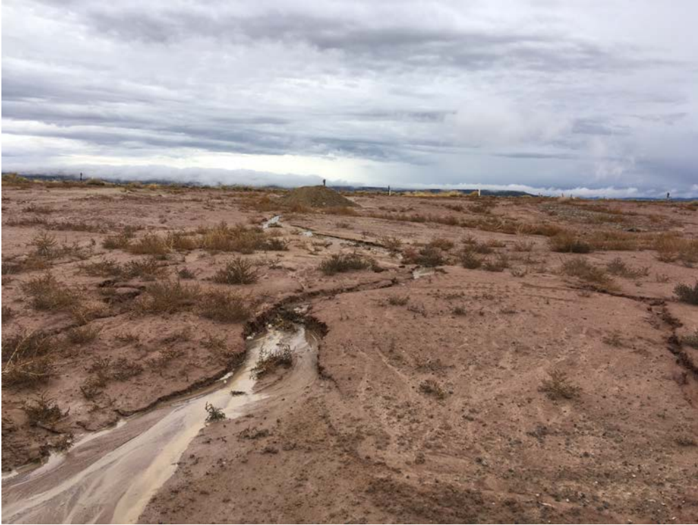
Photo 21: LTP, top surface rilling on east/southeast area
