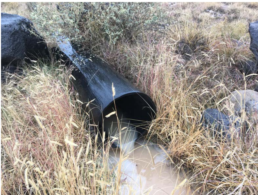
Photo 8: LTP, water draining from downdrain outlet on west slope
