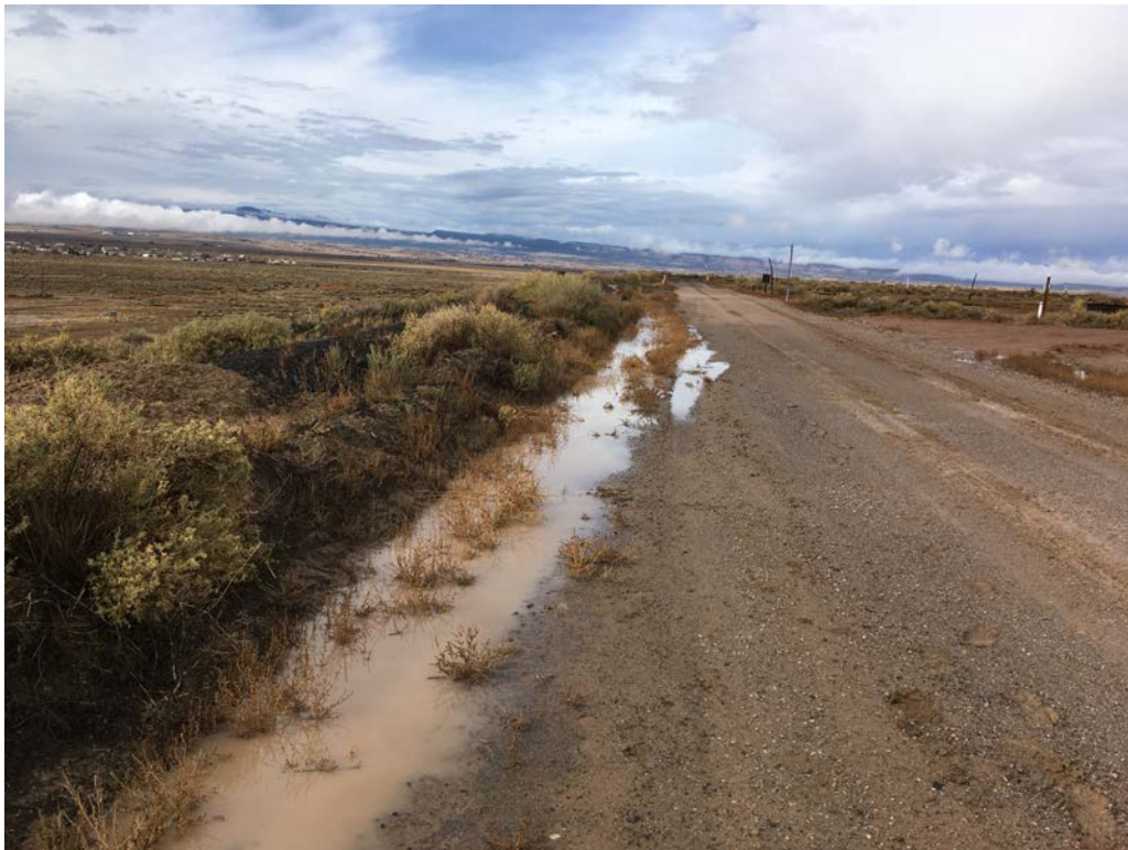
Photo 12: LTP, ponded water along crest road of south side slope
