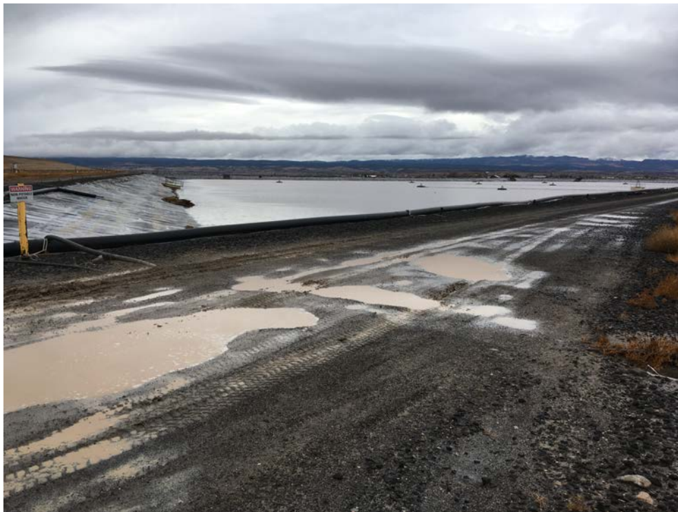
Photo 24: EP-2, ponded water along the access road and crest of the north embankment
