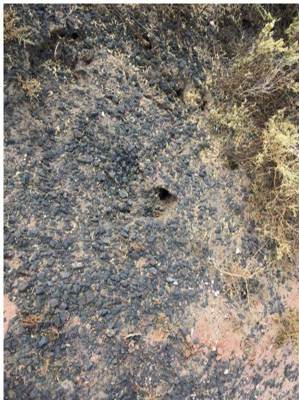
Photo 13: LTP, animal burrow on crest of south slope
