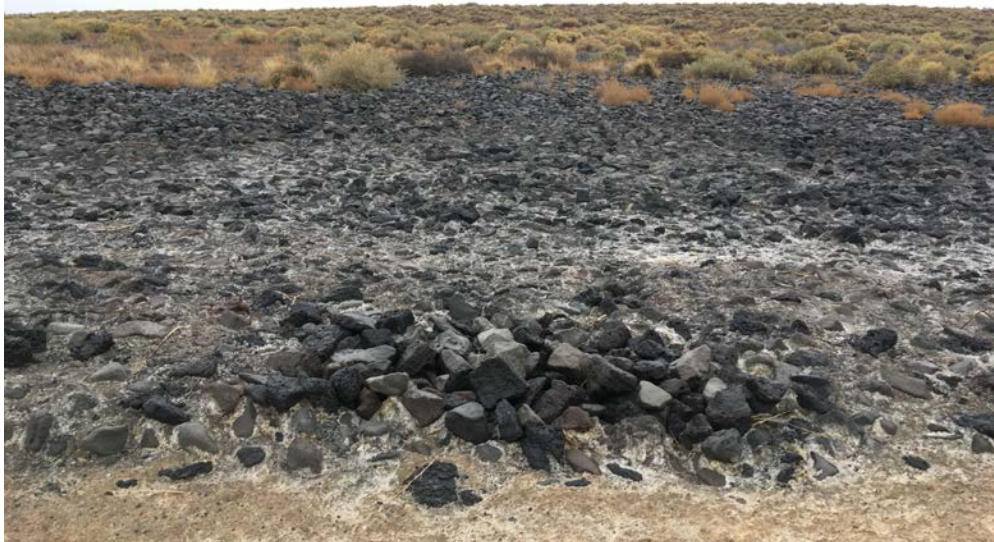
Photo 2: LTP, precipitate build up along downstream toe of north side slope
