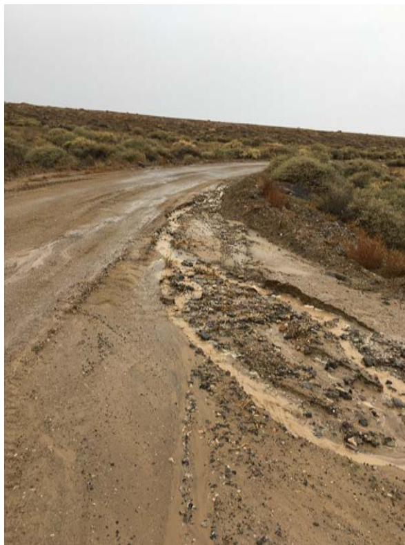
Photo 5: LTP, rilling along the side of the access road on north slope
