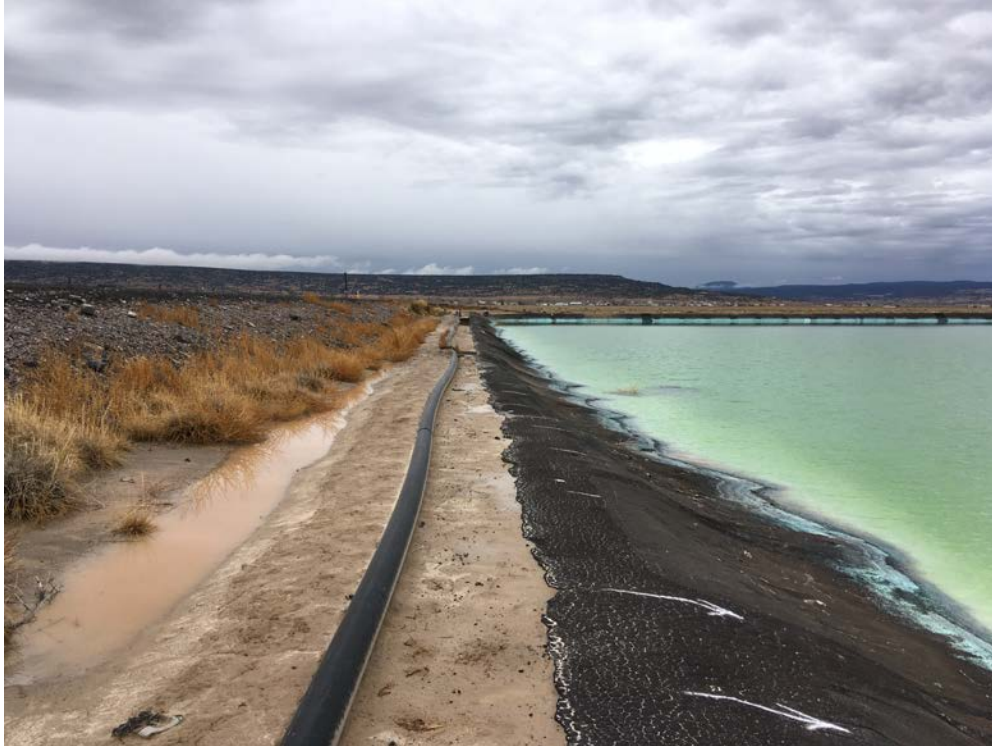
Photo 23: EP-2, ponded water along ridge at the toe of the west side slope of EP-2 and crest of east side slope of the east collection pond
