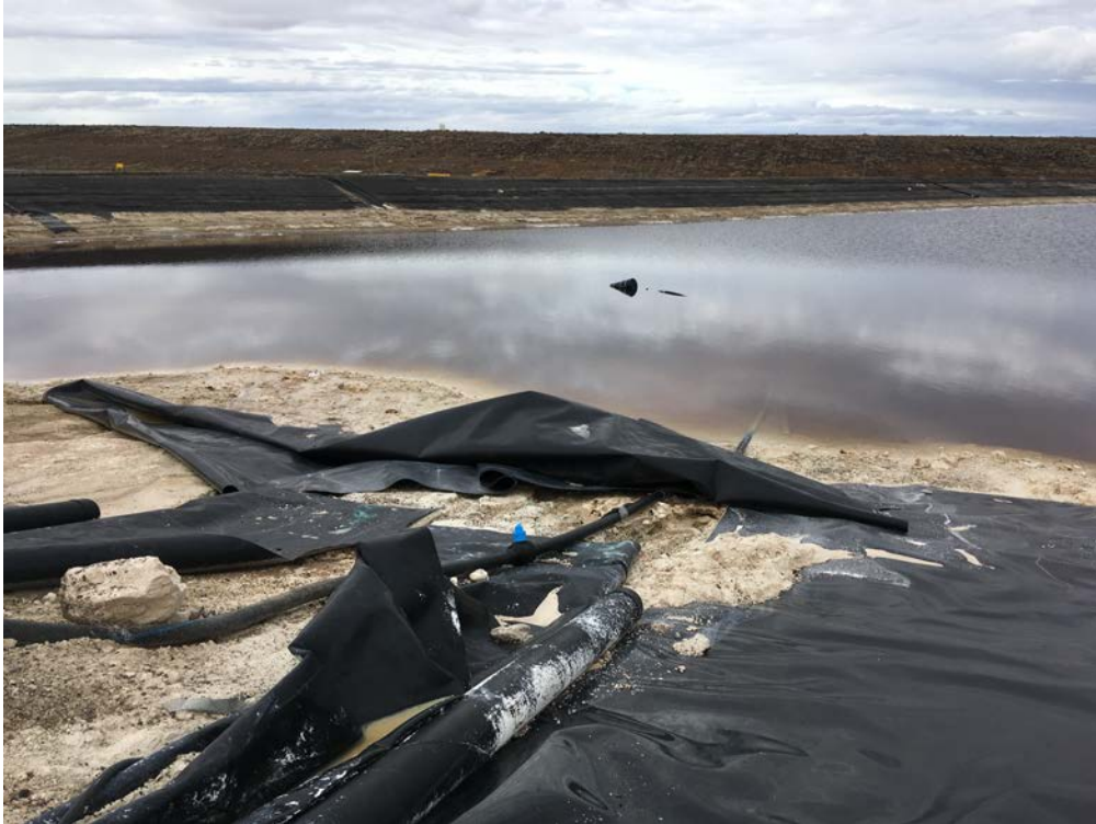
Photo 32: EP-1, location where WCP sediment being deposited to EP-1 along south embankment
