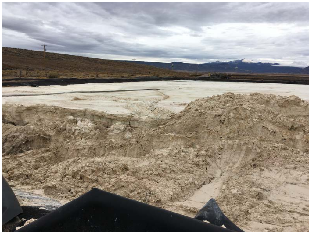
Photo 22: West collection pond, drained and some sediment removed from west end of pond
