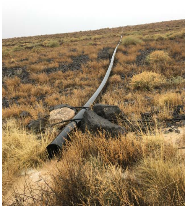
Photo 4: LTP, down drain outlet on north side slope
