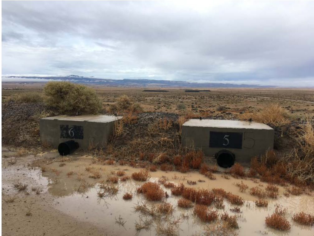
Photo 11: LTP, water ponded on west crest in front of downdrains 5 and 6 with water pooled in front. Water is not entering the inlet.
