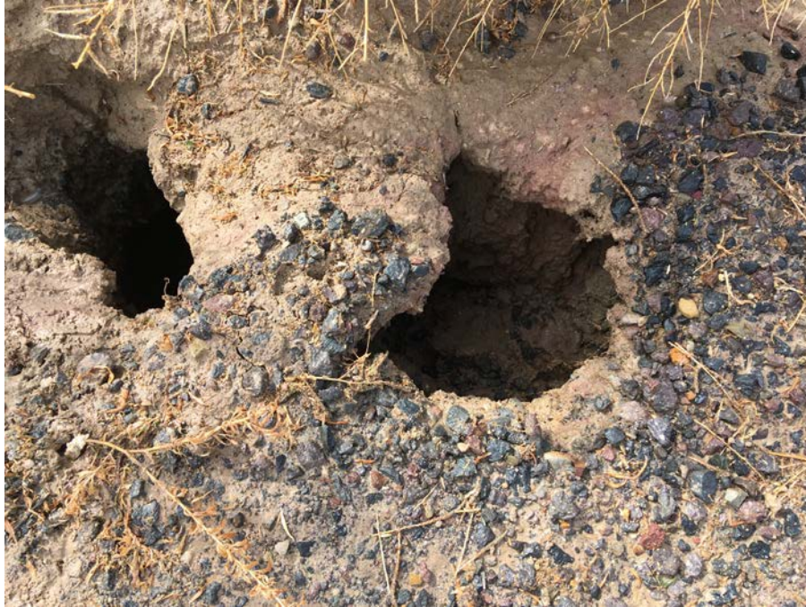
Photo 15: LTP, sinkhole near downdrain #11 on outer edge of south embankment crest
