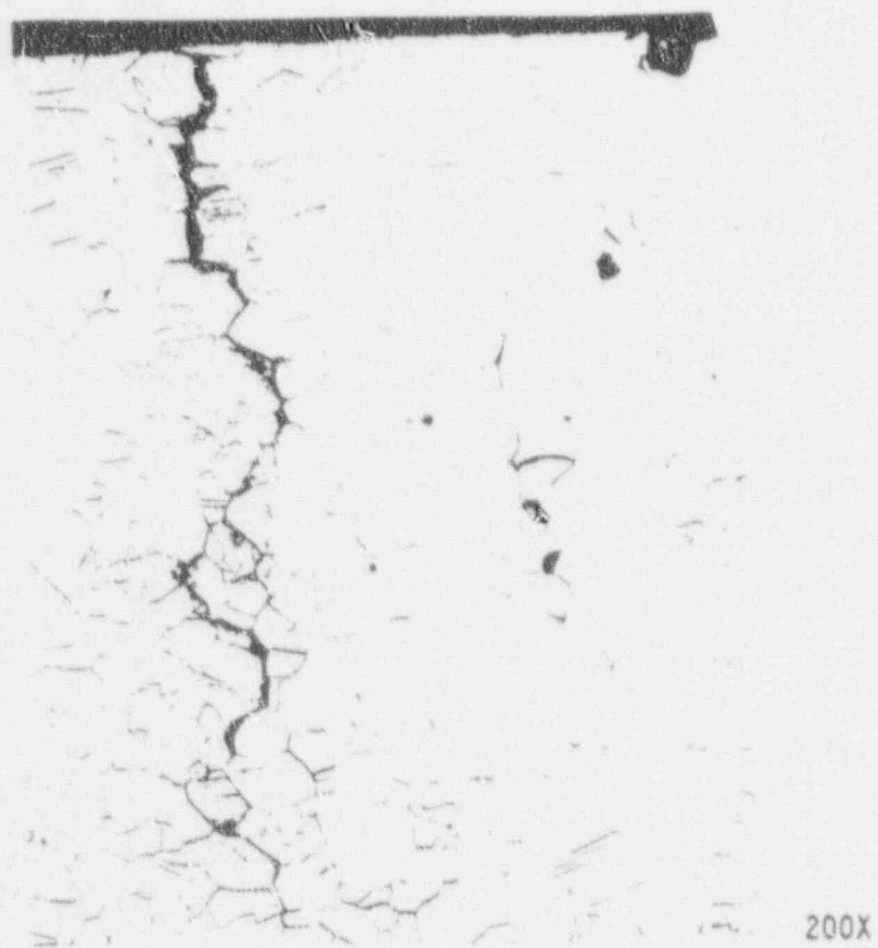
Figure 10-1 Sketch of a metallographic cross section through secondary support plate crevice cracks in Tube 543-4. A typical crack micrograph is also shown.
