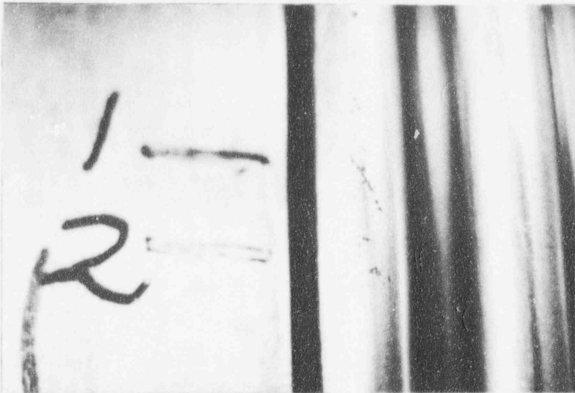
Figure 21. Test I-5-SCT. Specimen C-6-2 Showing Pretest Cracks.
