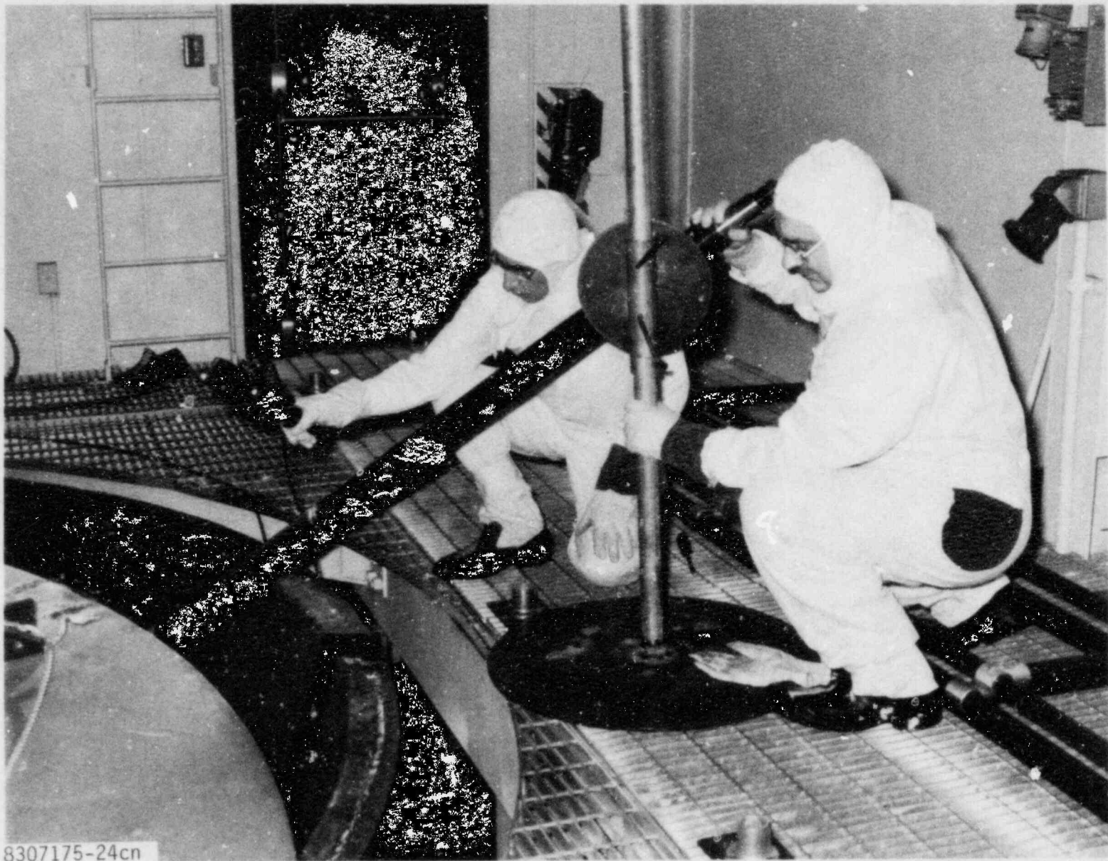
FIGURE 7. Observing Top of Steam Generator With a Multi-Jointed Periscope
