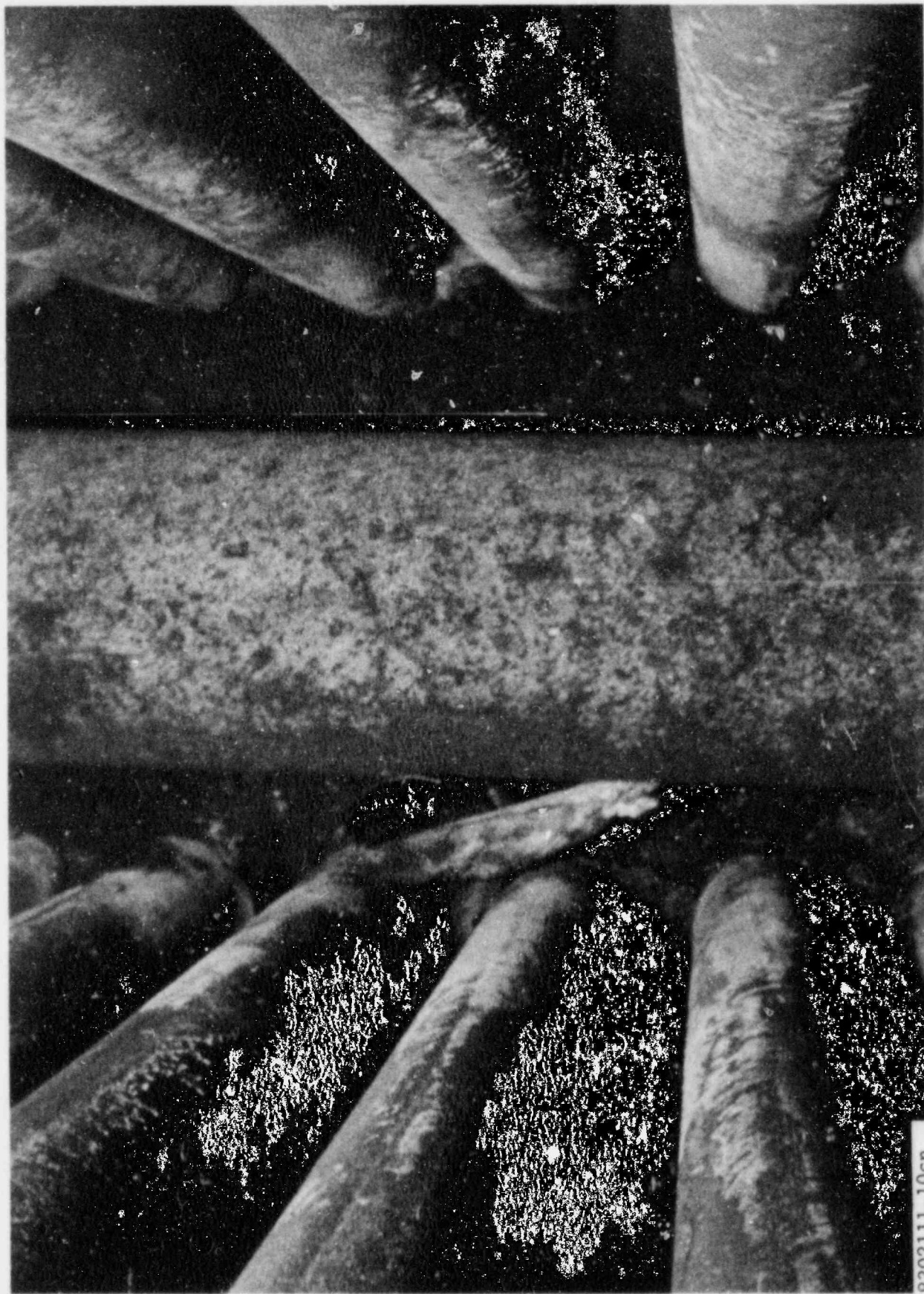
FIGURE 10. Close-Up View of Tube Sheet/Blowdown Pipe Region Around Tube Columns 75-80
