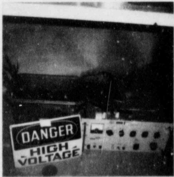
Figure 14. Setup for the Treeing Test
