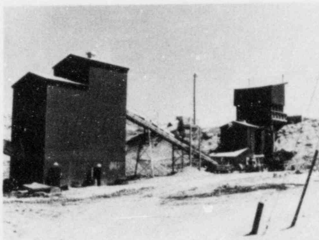
Uranium ore is fed through these primary and secondary crushers prior to processing at the Petrotomics Uranium Mill at Shirley Basin, Wyo.
