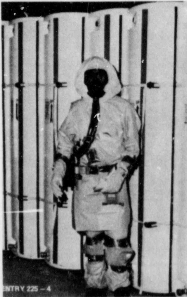
Close surveillance by NRC of the cleanup operations at Three Mile Island Unit 2 continues. This worker in protective clothing is standing in front of tanks containing water as shielding against radiation from contaminated areas inside the reactor containment building.
