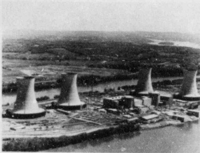
Unit 1 of the Three Mile Island nuclear power plant (Pa.) has been shut down since the accident at Unit 2 in March 1979. Possible restarting of the reactor has been the subject of a special proceeding. The Unit 1 reactor is housed in the building at the center-left and the unit includes the two cooling towers at the left.
