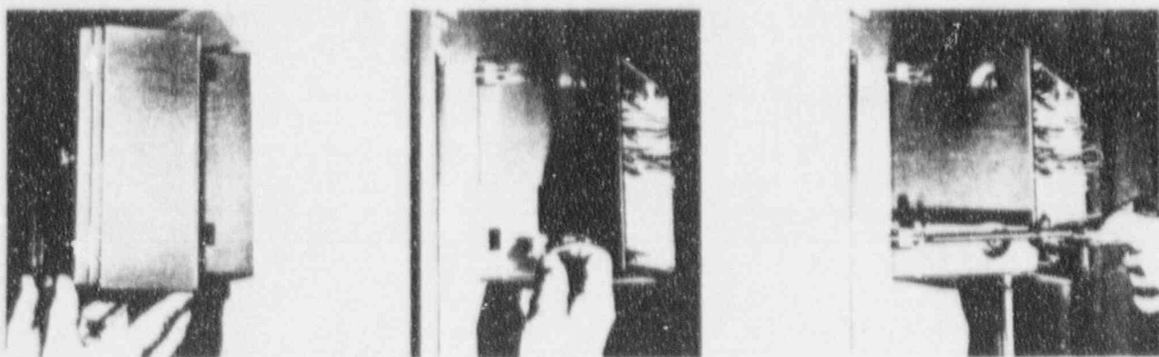
Fig. 1.2. Installation of a RHGX case in a panel (790900, 796898, 790899)
