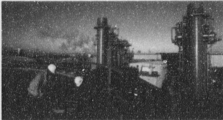
In March 1995, the San Jacinto Steam Electric Station began supplying steam to DuPont's La Porte chemical complex and low-cost electricity to HL&P customers.
