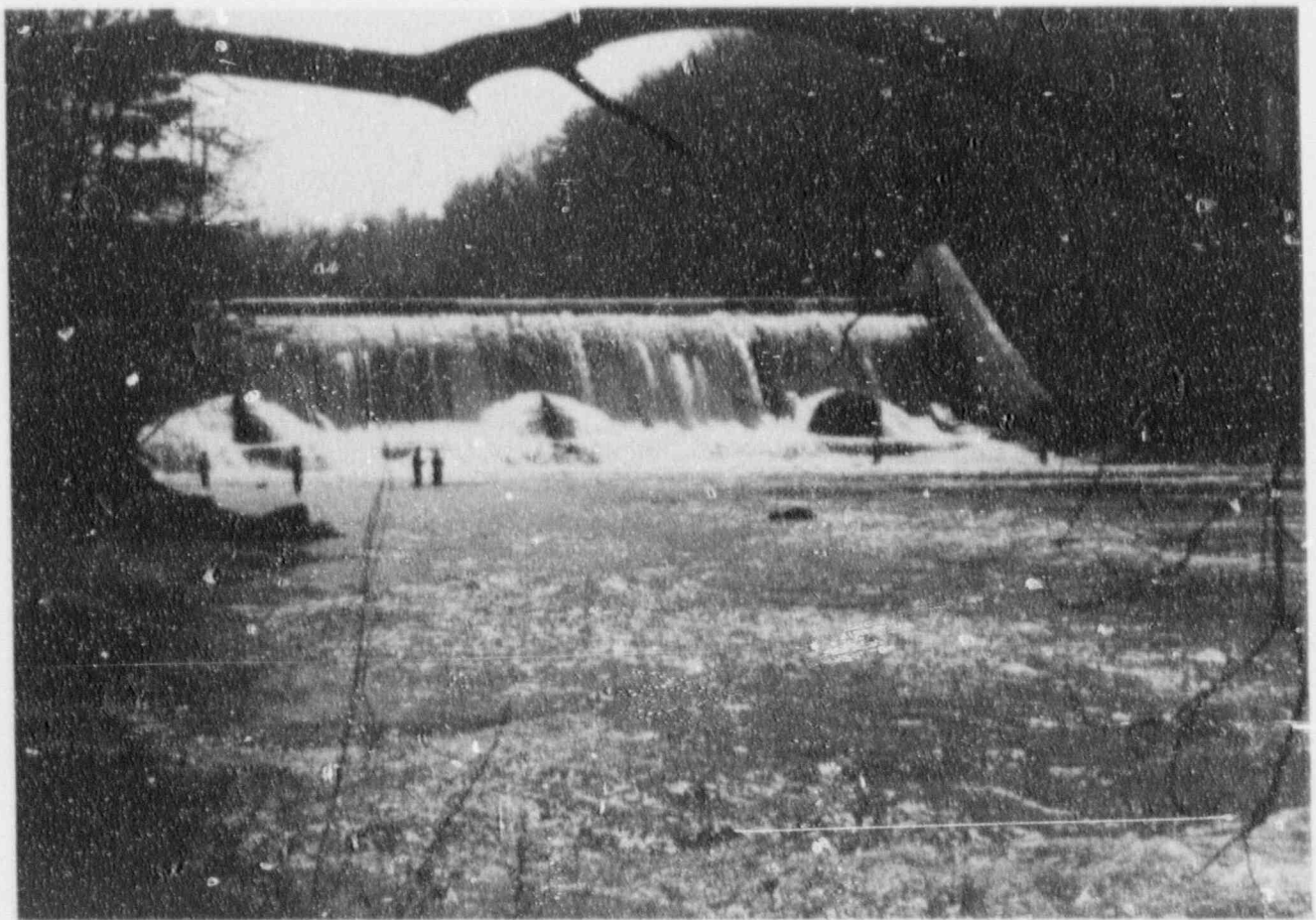
Springville Dam on Cattaraugus Creek
