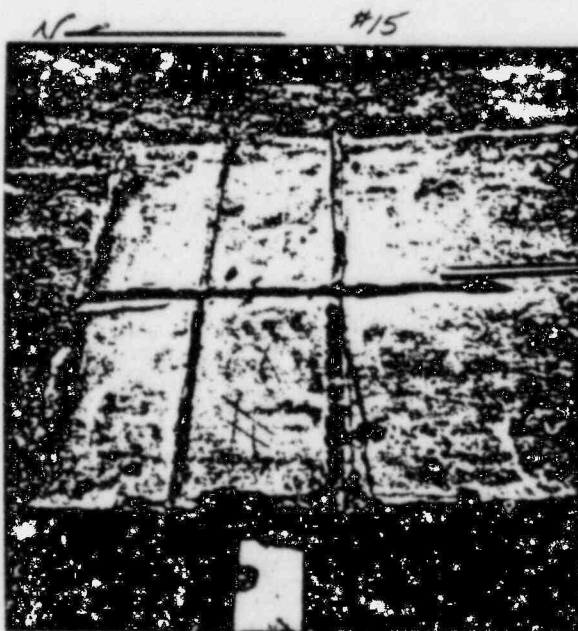
6/29/83 RATE No. 2 (NORTH END) CONCRETE CUT "H" PATTERN LEAD WOOL/EXP. METAL BULKHEAD 4 GROUT NIPPLES FOR WOOD RATE
