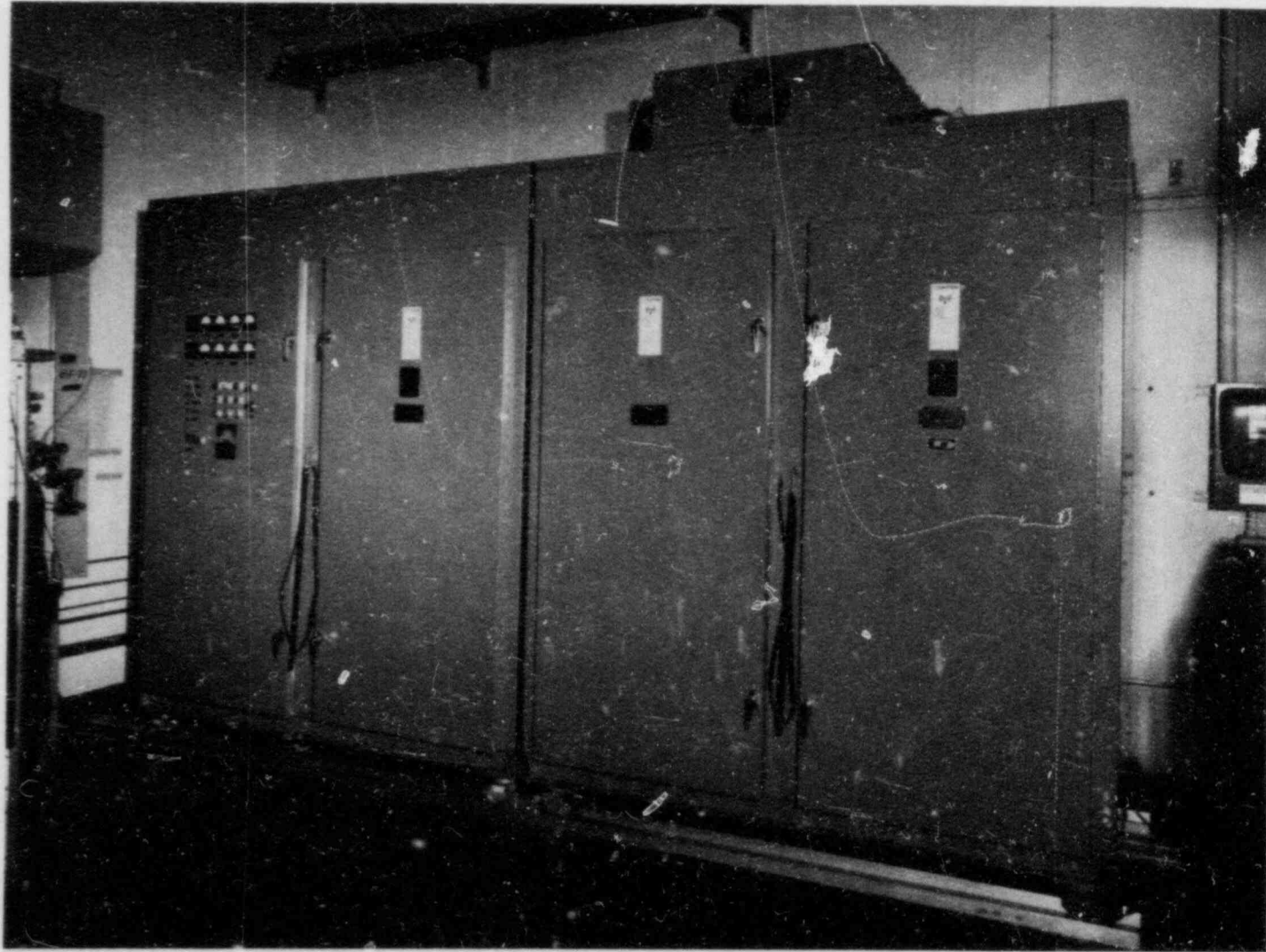
Fig. 17. 250-kW rf induction generator at ORNL.
