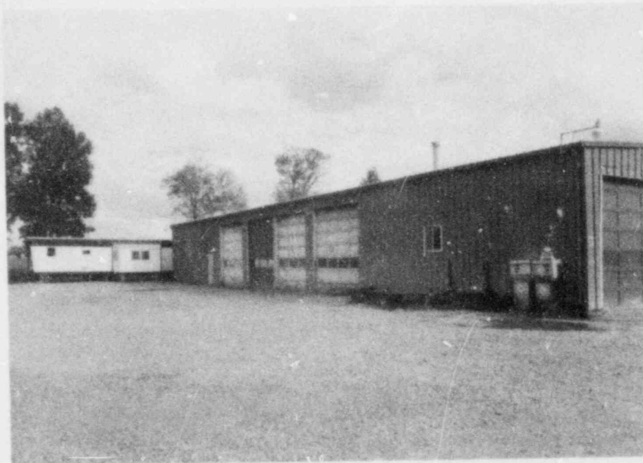
Figure 4. Shelwell Building 1 and office trailer.
