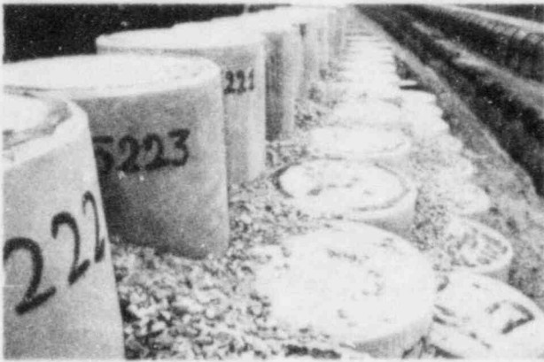
a. Along the perimeter of the area, the blocks are stacked in a stepped arrangement to provide stability and to give the final tumulus the shape of a sloping mound,
