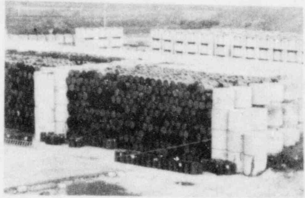
b. Metal drums containing low-level wastes which have been placed inside the "compartments" formed by rows of concrete blocks at the Centre de la Manche, France.
