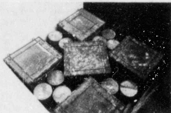
a. Intermediate-level, nonirradiating wastes are lowered by crane into compartments in successive layers. After each layer is placed, it is backfilled with concrete.
