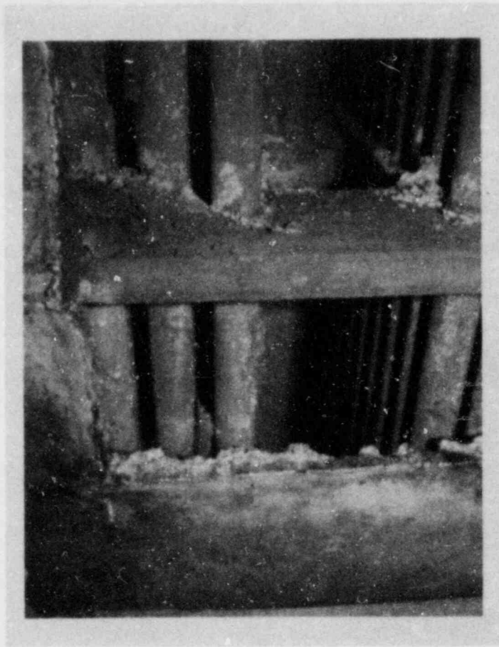
FIGURE 42. Condition of First Support Plate at Penetration 1 Before Shipment
