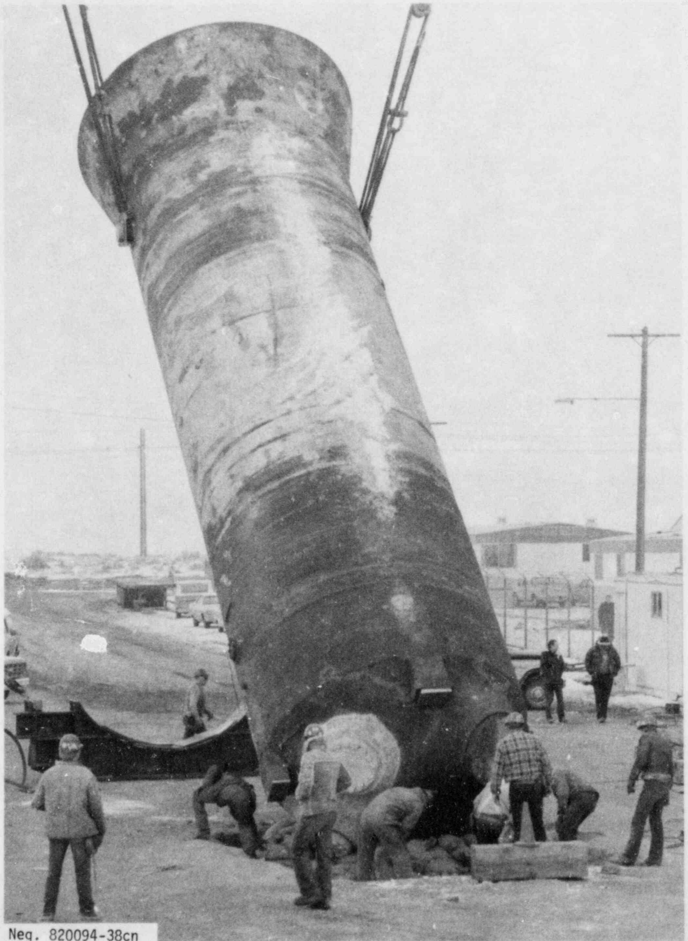
FIGURE 17. Sand Bag Pit for Upending Generator
