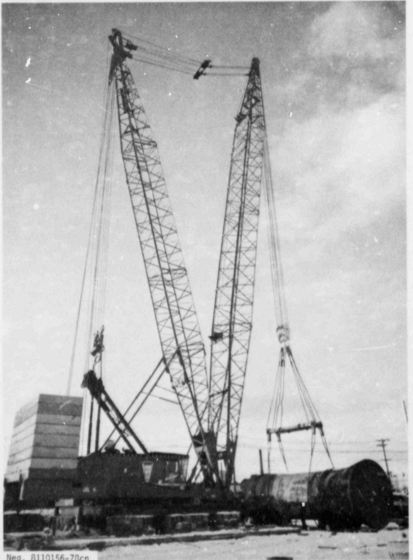
FIGURE 13. Manitowoc 4100 Ringer Crane
