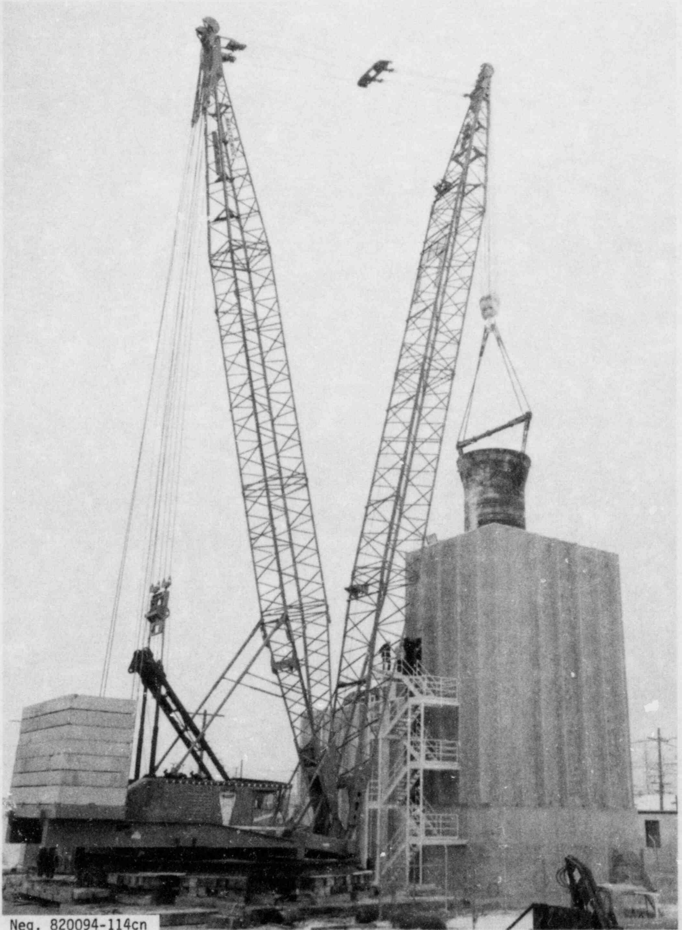
FIGURE 19. Lifting Generator Into SGEF
