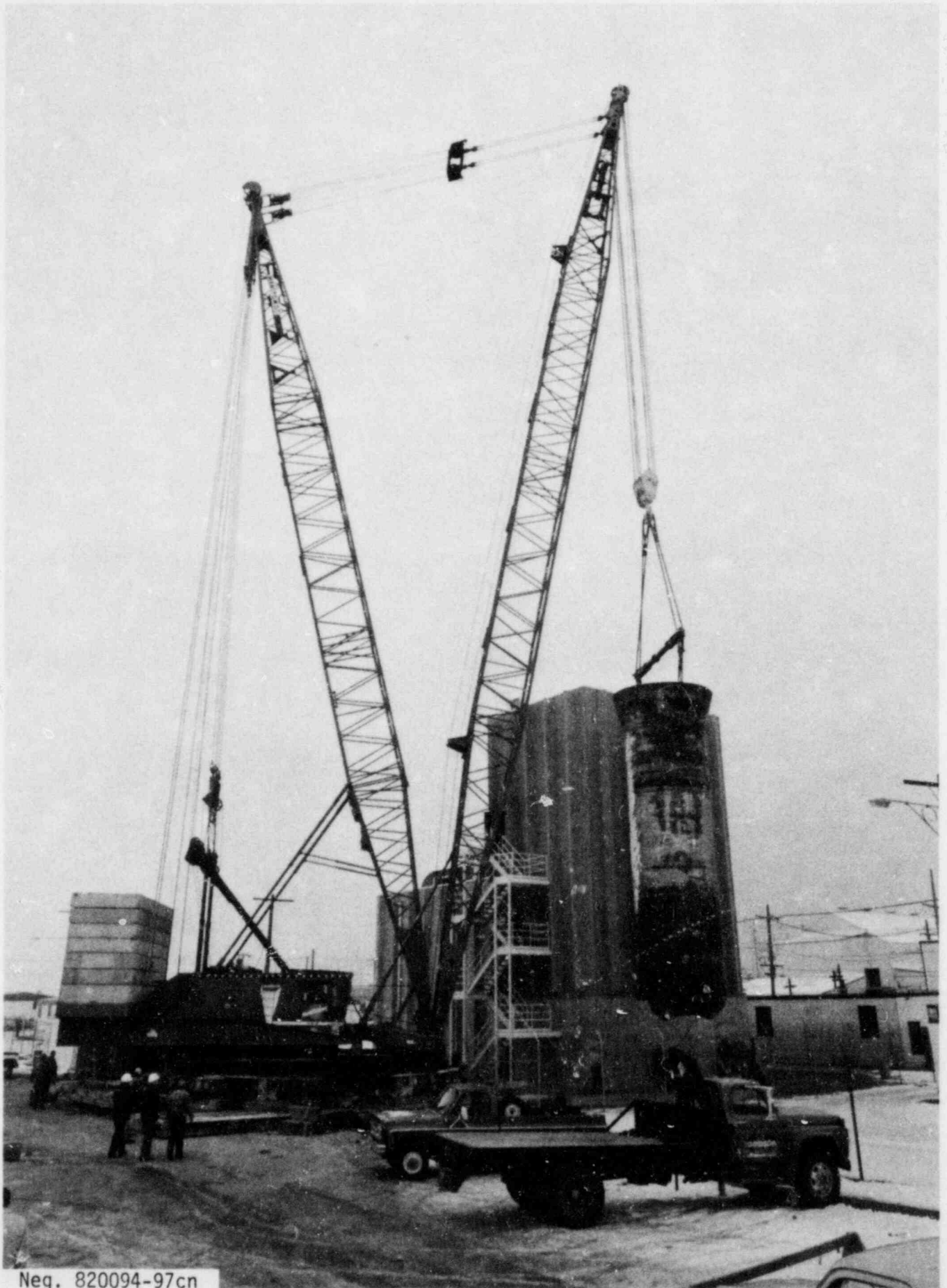
FIGURE 18. Lifting Generator Into SGEF
