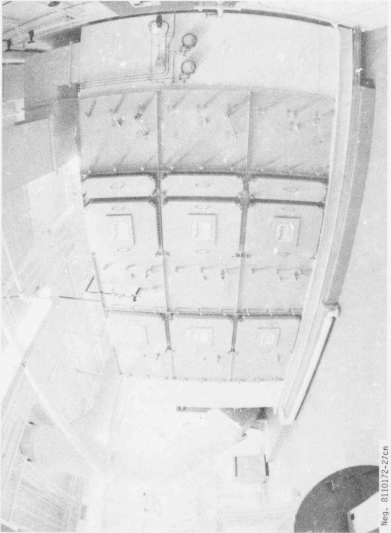
FIGURE 12. HEPA Filter Bank in Equipment Room
