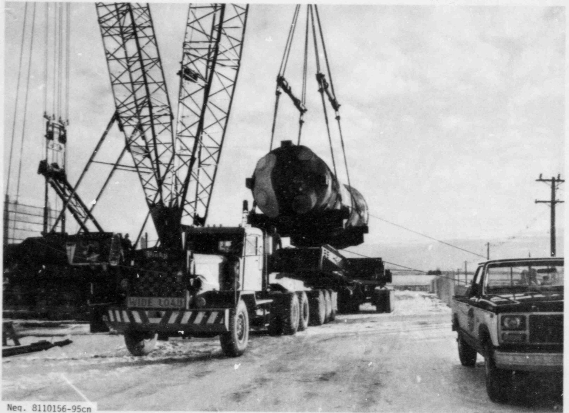
FIGURE 15. Lifting Generator Onto Trailer
