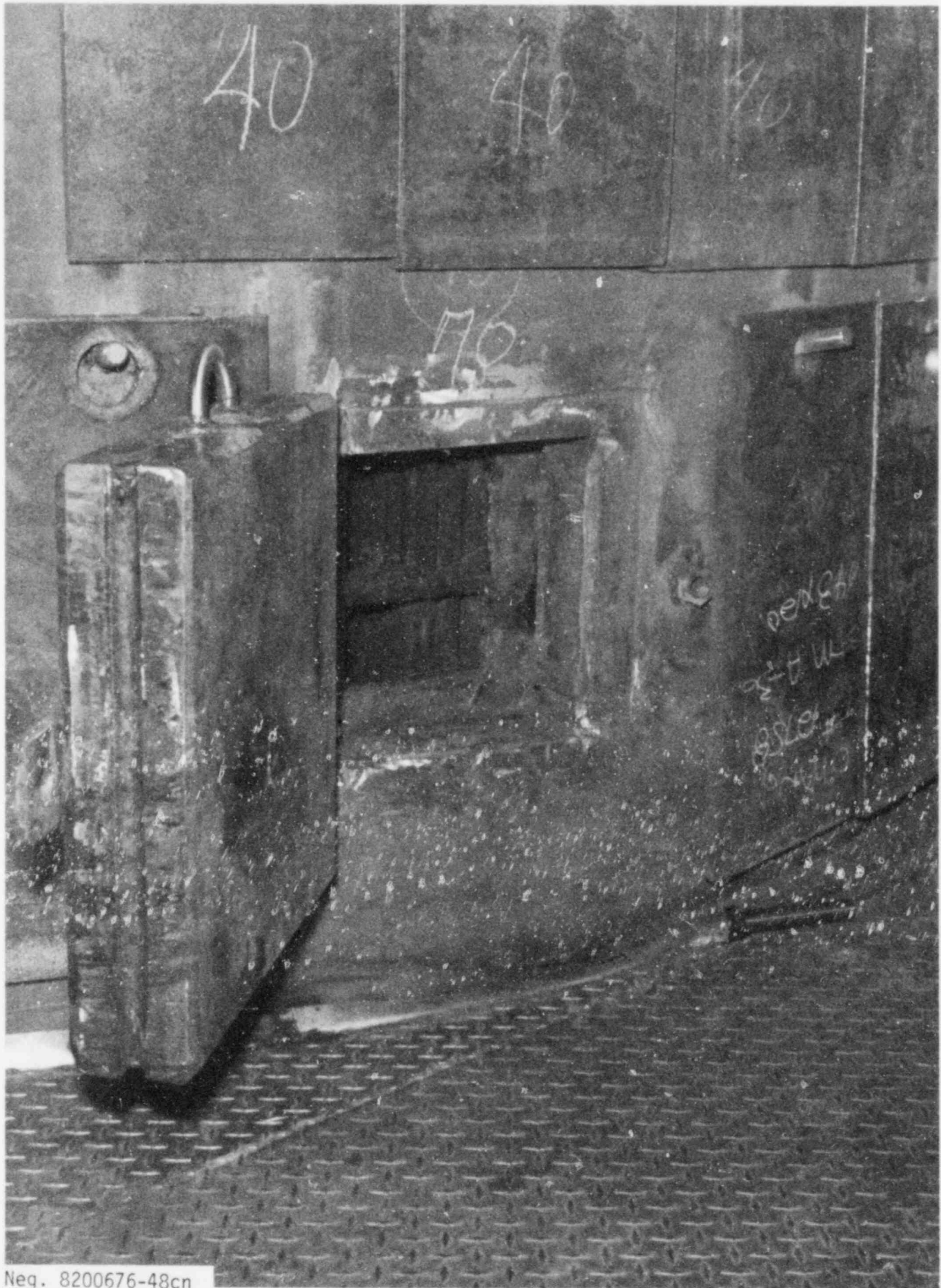
FIGURE 39. Penetration Access in SGEF at Cut 1
