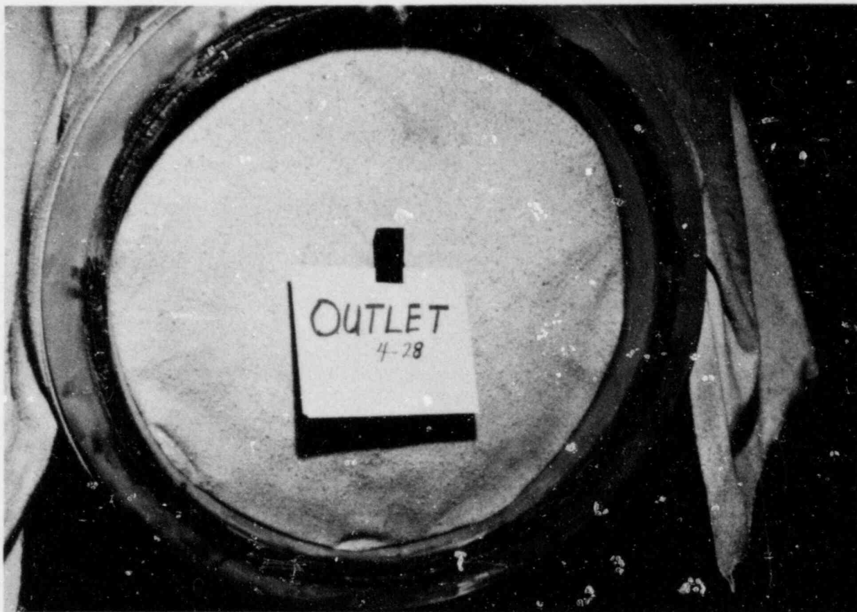
FIGURE 22. OUTLET NOZZLE DURING REPAIR WELDING - BUILDUP OF WELD LIP.
