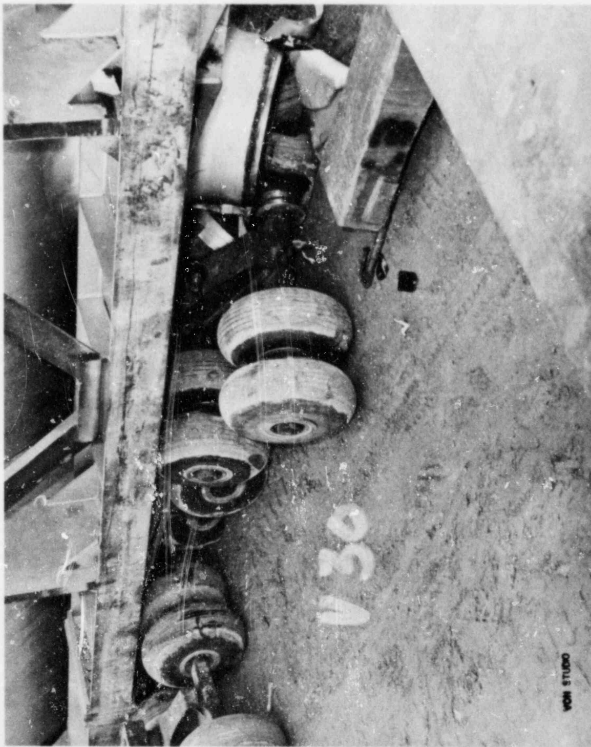
FIGURE 10. OUTLET NOZZLE RESTING ON DOLLY WHEEL RIM WITH TIRES AND AXLE EXTENDING INTO NOZZLE BORE - VIEW 3.
