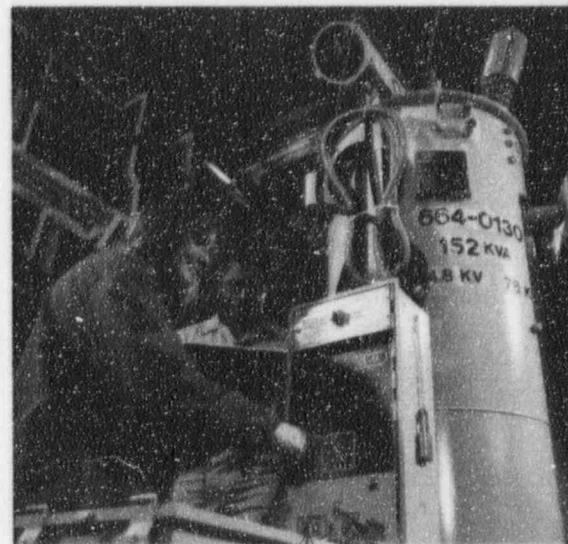
Detroit Edison's Craig L. Smith, engineering technician, shows Wayne State University engineering student Patricia A. Kohlman a voltage regulator designed by company employees and Cooper Power Systems of Waukesha, Wis. The new standardized regulator improves service reliability and is less expensive to produce.
