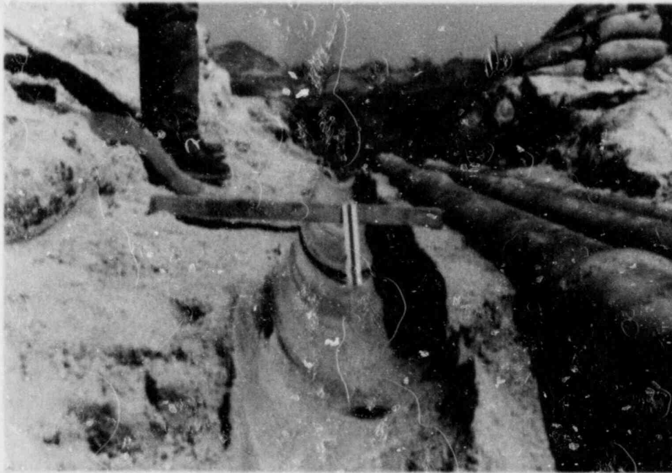
BACKFILL BETWEEN AND BENEATH PIPES SUBSEQUENT TO PIPE REMOVAL
