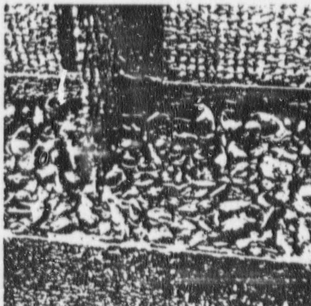
Figure 1. Asiatic clams growing on the plant side of influent screens. Clam-trol CT-1, unlike halogen or screening methods, controls both larval and adult clams.
